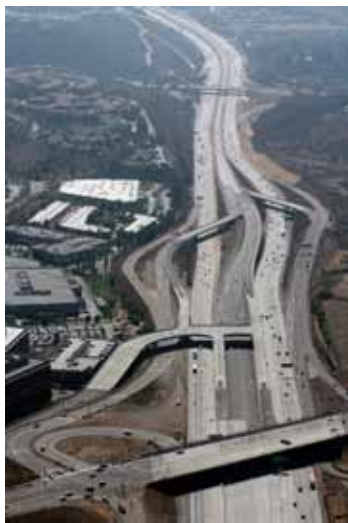
Aerial view of Southern California I-15 HOT lanes. (Photo courtesy of California Department of Transportation, District 11.)
