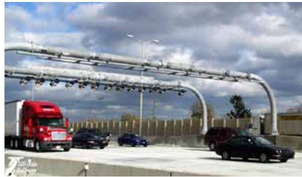
Open road tolling on the Illinois Tri-State Tollway. (Photo courtesy of Illinois Tollway.)
