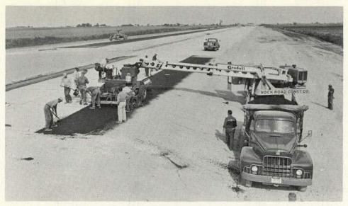
Figure 19. Paving shoulders on rigid tangent.
