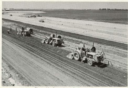
Figure 36. Processing embankment soil.
