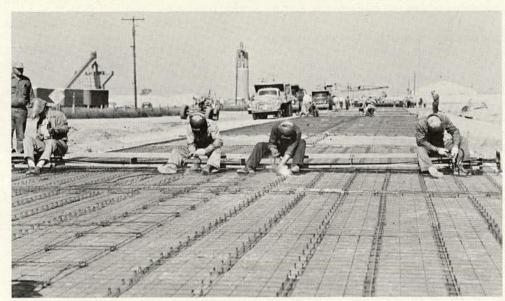
Figure 104. Placing fabric in 21/2- and 31/2-in. pavements on Loop 2.
