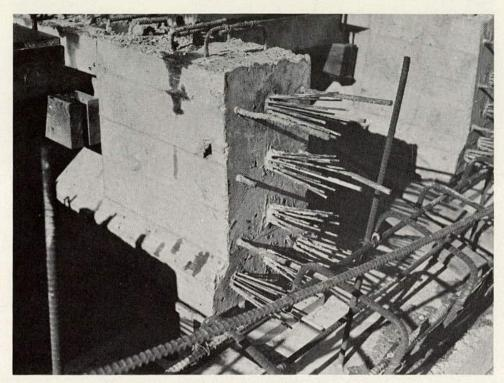
Figure 131. End of post-tensioned beam, Bridge 5B.
