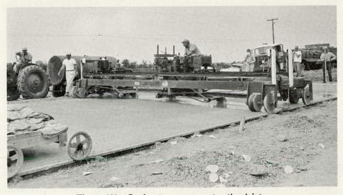
Figure 109. Sawing transverse contraction joints.
