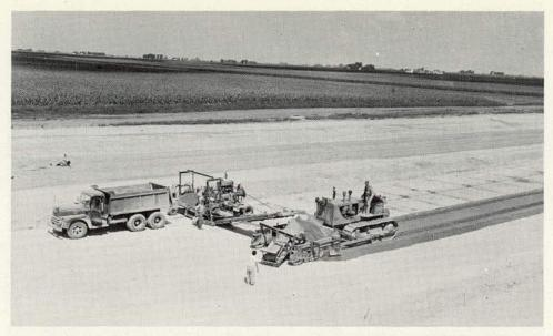
Figure 54. Placing sand-gravel mulch on embankment from outside shoulder.
