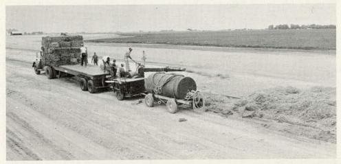
Figure 108. Placing straw for curing concrete.
