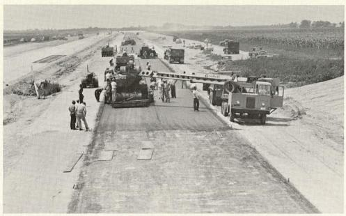
Figure 96. Constructing initial layer of binder course; second machine in position to pave other lane.
