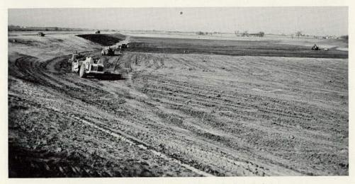
Figure 35. Restoring borrow pit to farmable condition.
