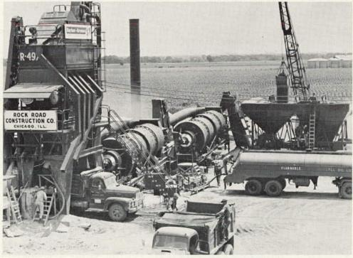
Figure 92. Automatic batch-type plant used to produce binder course mixture; dryers in tandem.
