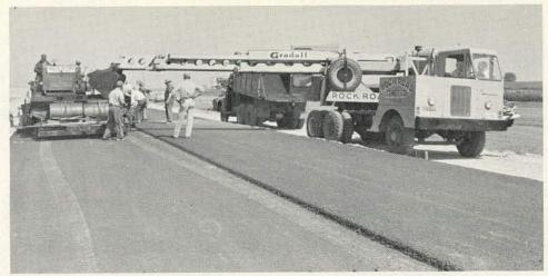
Figure 95. Depositing mixture in paver from outside shoulder.
