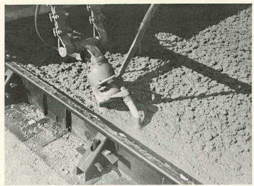
Figure 106. Vibrator on concrete spreader.
