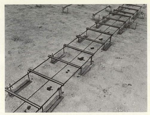
Figure 18. Transverse contraction joint assembly.
