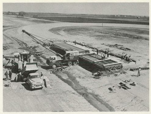
Figure 137. Casting bridge slab.
