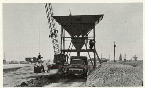
Figure 83. Batching aggregate for gravel base course, special.
