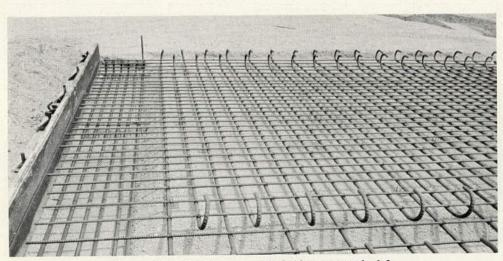
Figure 121. Reinforcement in bridge approach slab.
