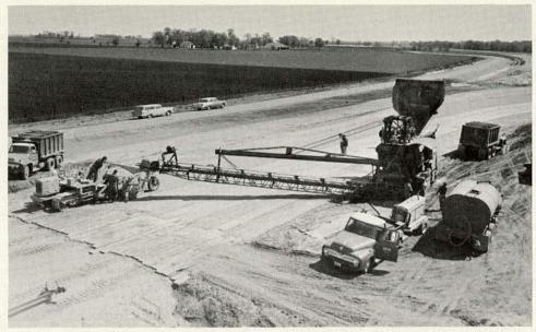
Figure 75. Depositing and spreading crushed stone base; planks in transition for equipment crossing.
