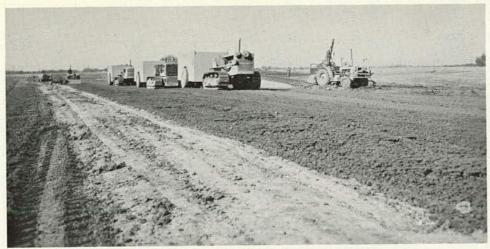
Figure 37. Compacting embankment soil.
