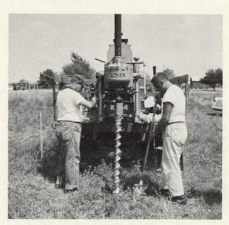
Figure 29. Drill rig in borrow pit.
