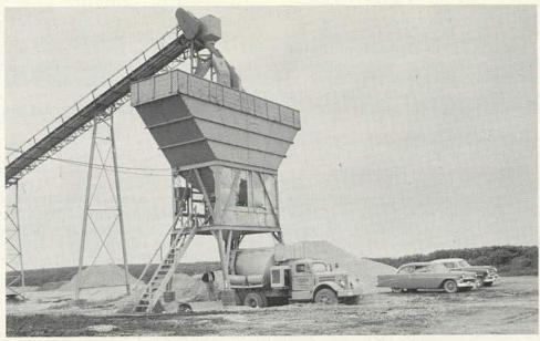
Figure 84. Batching aggregate for cement-treated base course.
