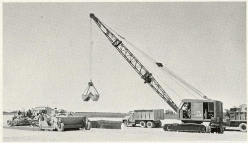
Figure 55. Placing additional material for subbase construction from outside shoulder.
