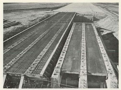
Figure 129. Prestressed concrete beam bridges showing slab reinforcement, recessed keys and extended stirrups.
