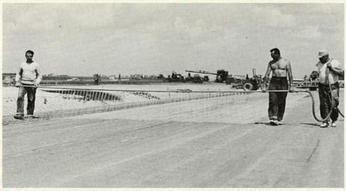
Figure 56. Adding water for compaction of subbase.
