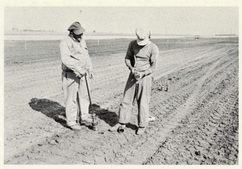
Figure 41. Obtaining soil sample for field density.
