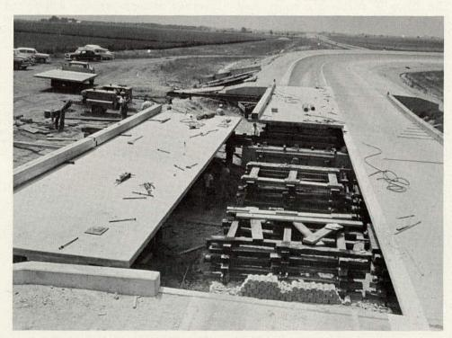
Figure 140. Jacking bridges 9A and 9B into place on existing bearings.
