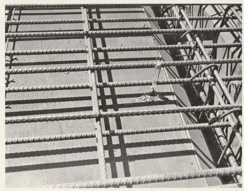
Figure 133. Reinforcement in concrete beam bridges; thermocouple on steel.
