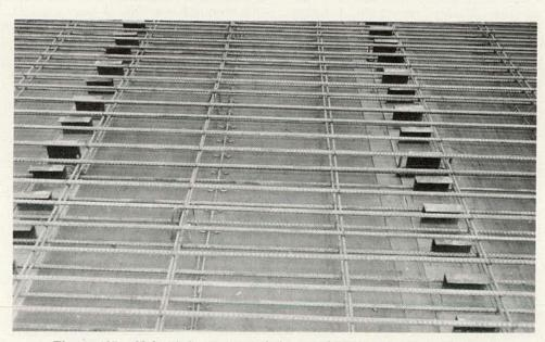
Figure 125. Slab reinforcement and channel shear connectors in composite steel beam bridges.
