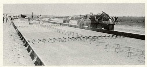
Figure 105. Wetting subgrade ahead of paving; transverse and longitudinal joint assemblies in place.
