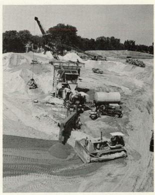
Figure 53. Mixing plant for stabilizing subbase material.
