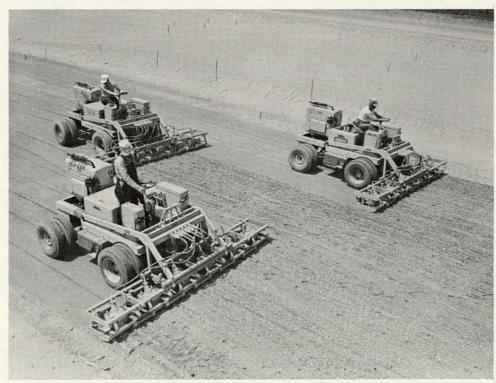
Figure 57. Compacting subbase.
