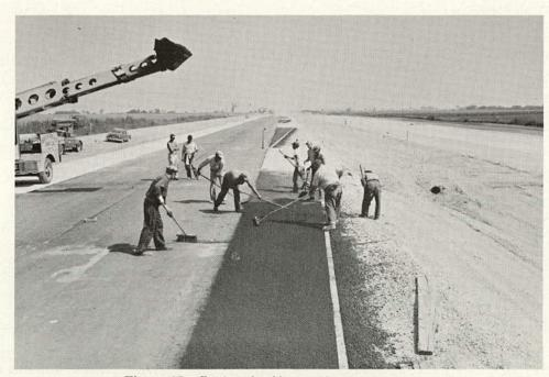
Figure 97. Paving shoulders on flexible tangent.
