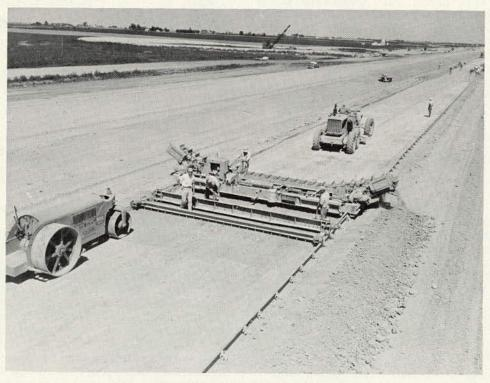
Figure 39. Subgrading top of embankment.
