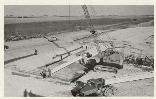
Figure 130. Erecting precast prestressed concrete beams.
