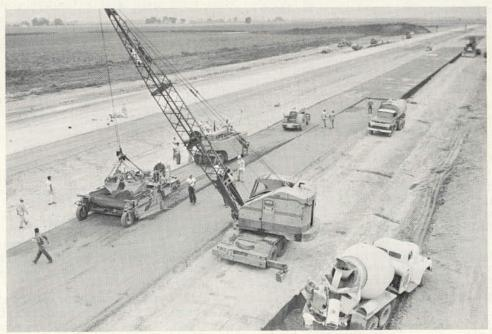
Figure 86. Constructing cement-treated base course.
