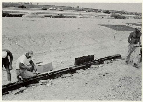
Figure 111. Preparing concrete test specimens.
