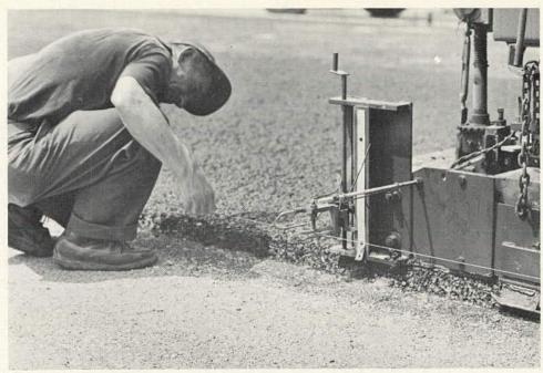
Figure 101. Device on paver for following guide wire.
