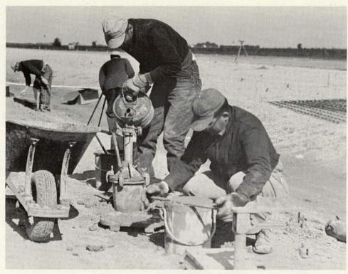
Figure 110. Testing plastic concrete.
