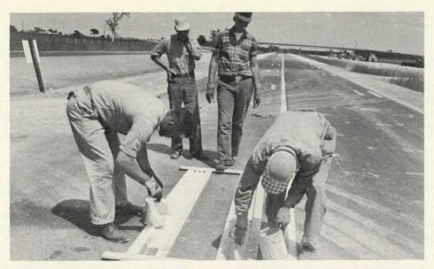
Figure 45. Guide lines on Loop 2 were painted by hand because the weight of paint striping equipment exceeded that of the test vehicles.
