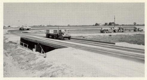
Figure 4. Test bridge site. Four 50-ft span bridges are built on common substructure.
