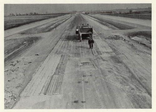
Figure 43. Pierced steel-plank mats were used successfully as a temporary riding surface over damaged areas pending more permanent repairs.
