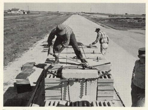
Figure 47. Maintenance forces assisted in loading and load banding on test vehicles.
