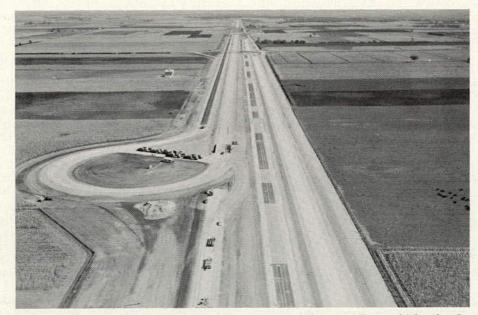
Figure 2. View of Loop 5 (at left) and a portion of Loop 2. Test vehicles for Loop 5 are parked in the crossover road in the turnaround.
