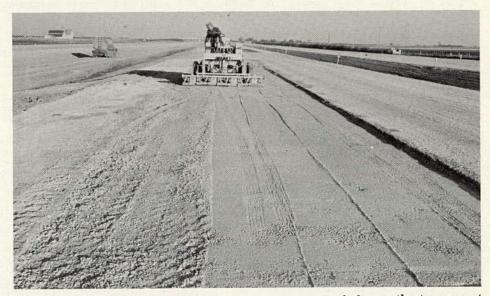
Figure 37. A multiple-pan vibratory compactor was used frequently to compact crushed stone used as a base in deep patches.
