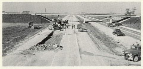
Figure 39. Many of the thinner pavement sections were excavated and rebuilt following their removal from testing. Here, an entire test section has been dug out prior to backfilling with crushed stone and surfacing with hot-mix asphaltic concrete.
