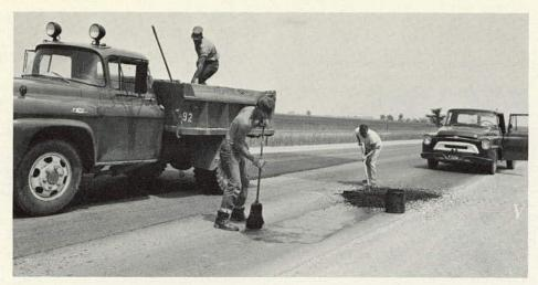
Figure 36. Project maintenance forces placing a skin patch consisting of an application of bitumen and pre-mixed bituminous patching material.
