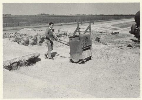
Figure 41. A hand-operated vibratory roller was used to compact crushed stone when excavated areas were too small for conventional compaction equipment.
