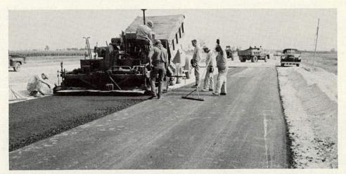
Figure 38. Many sections declared out of test were reinforced with a hot-mix asphaltic concrete overlay. Routine measurements and observations were continued on selected overlaid sections.
