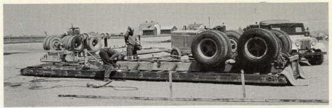
Figure 31. Welding crew rebuilding and reinforcing frame of a semitrailer that suffered fatigue damage as a result of constant operation under full load.
