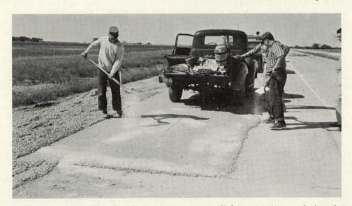
Figure 42. Traffic was allowed to operate over crushed stone prior to placing the surfacing. Calcium chloride was used to stabilize the granular material and reduce dust.
