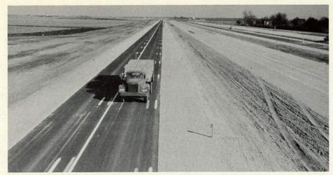
Figure 23. Guide lines were painted on left side of each traffic lane to assist drivers in maintaining proper transverse placement.
