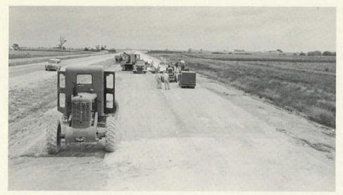
Figure 40. Manpower and equipment frequently were concentrated on small areas requiring maintenance in order to complete the work during the 5-hr traffic break.
