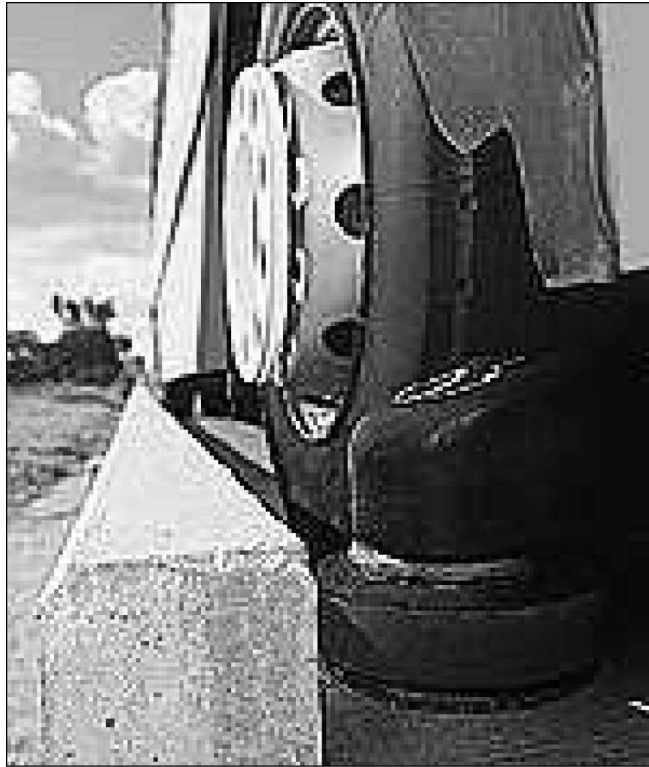
Figure 3: O-Bahn Guideway Section
