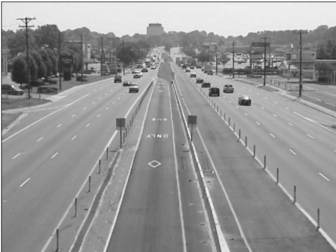
Figure 5: Western Terminus Showing Queue Jumper Lane
