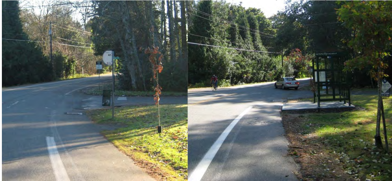
Figure 6-16. Before and After Construction of a Curb-Height Concrete Pad, with Ramp to Shoulder, and Shelter Installation (photos courtesy of Intercity Transit)
