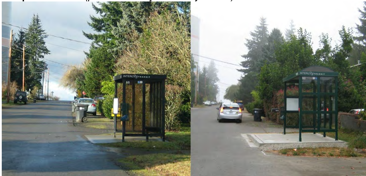
Figure 6-13. Before and After Construction of a Curb-Height Concrete Pad, with Ramp to Shoulder ( photos courtesy of Intercity Transit )
