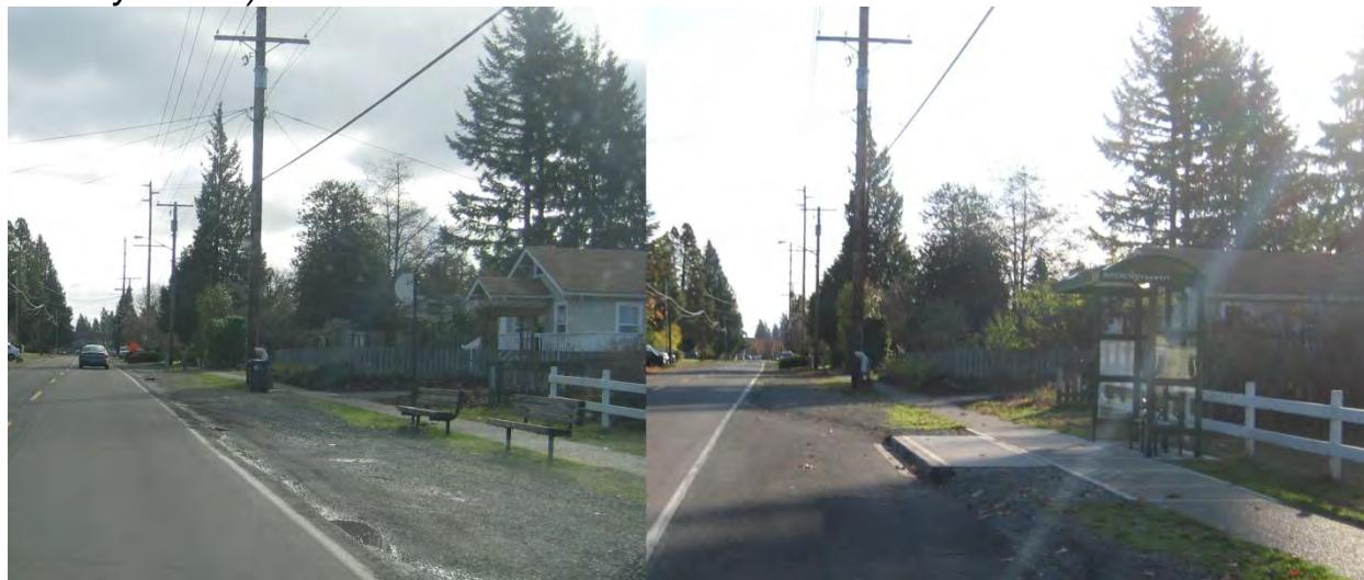
Figure 6-15 Before and After Construction of a Curb-Height Concrete Pad Extending from Sidewalk to Shoulder, and Shelter Installation (photos courtesy of Intercity Transit)
