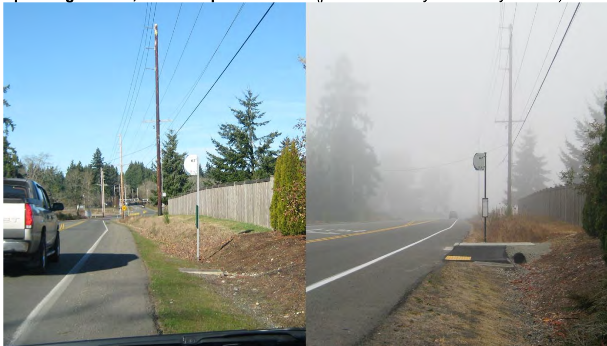
Figure 6-14. Before and After Construction of a Curb-Height Concrete Pad Spanning Culvert, with Ramp to Shoulder (photos courtesy of Intercity Transit)
