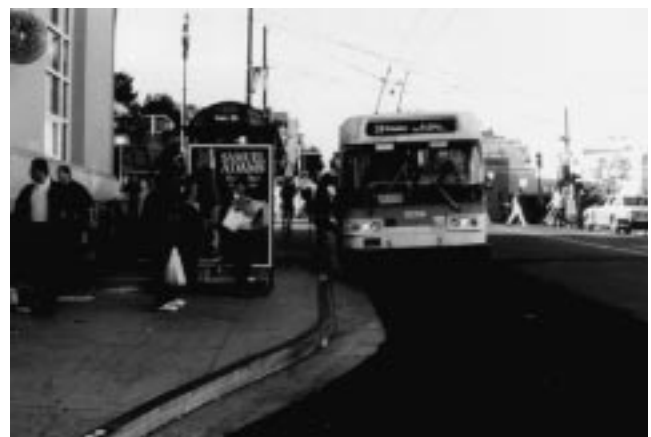
Figure 2-6. With the addition of bus bulbs, buses are able to load from the moving lane, and sidewalk circulation space has increased.
