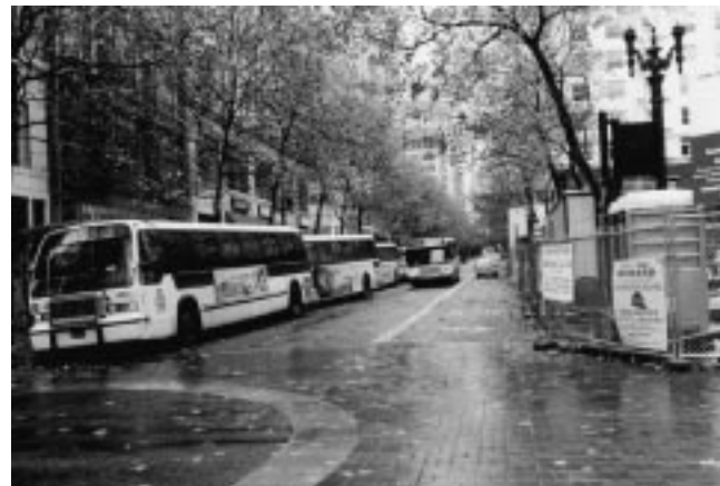
Figure 4-4. Bus priority lanes on the Portland Mall, Portland, Oregon.
