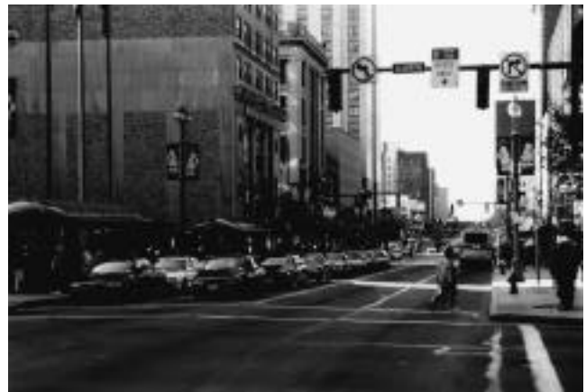
Figure 3-6. The dedicated bus-only curb lane is identified by signage at each intersection.
