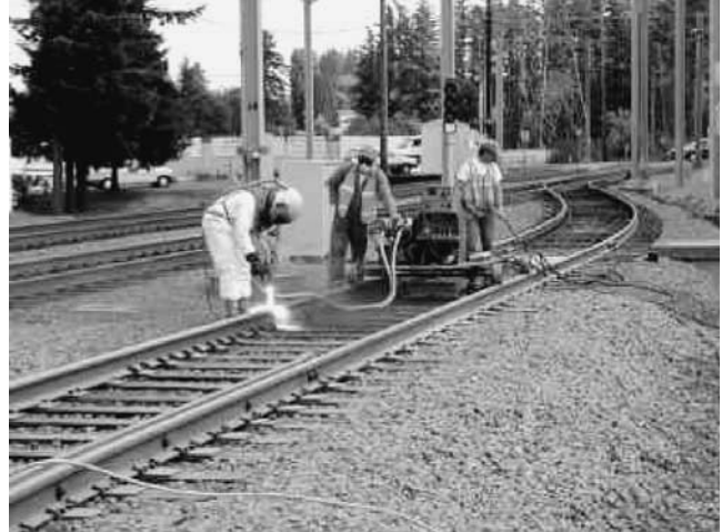
Figure 8. Application of coated film onto rail.
