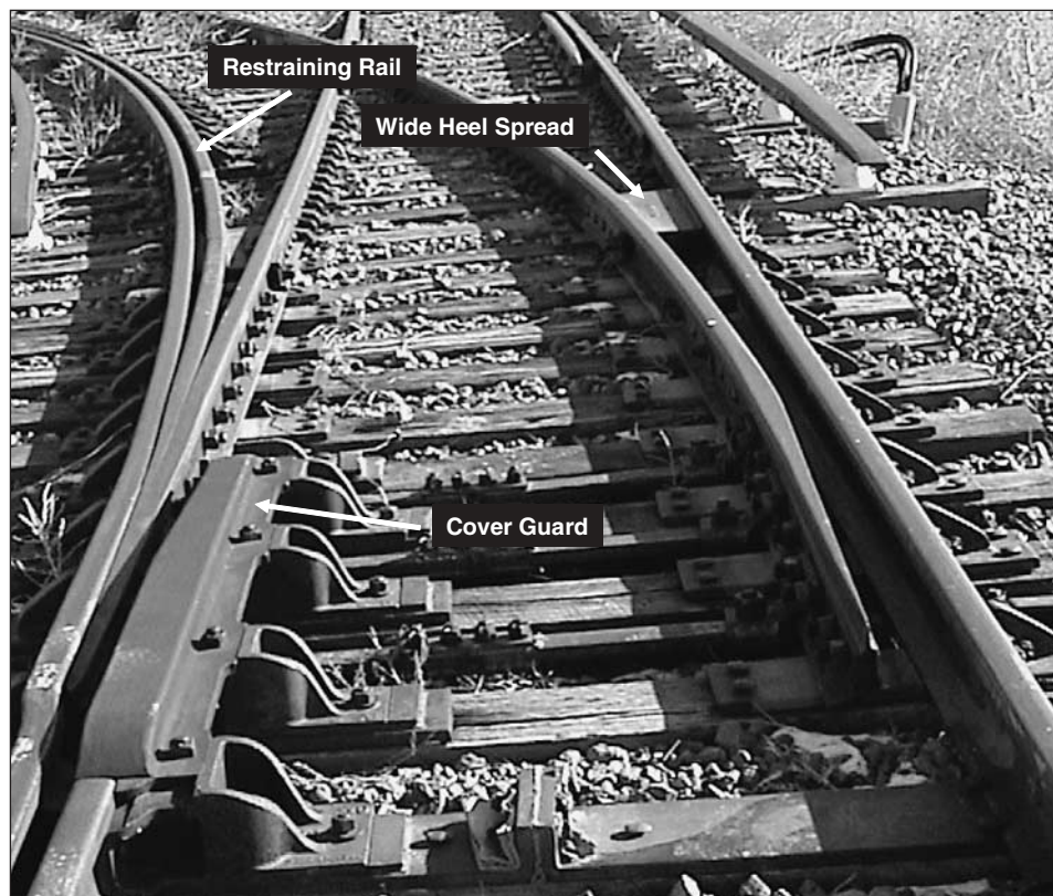
Figure 4. Typical guarded switch with cover guard.
