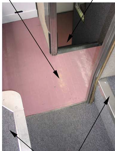
Stair-to-corridor transition landing 24" x 40"
