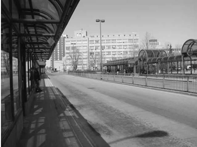
Figure 4. Barrier between opposing directions of travel at Ottawa Transitway station.
