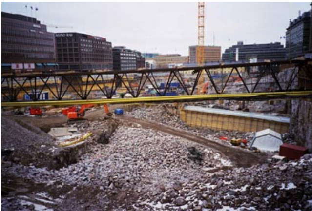
Figure 8. Kampii bus station under construction.
