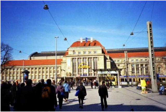
Figure 5. The majestic Promenaden Hauptbahnhof rail station and shopping mall.
