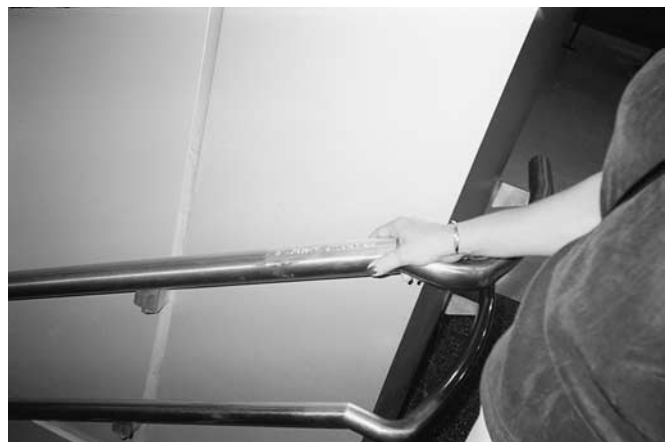
Figure 29 Braille etchings on handrails to help the visually impaired navigate the stairs in Santiago.
