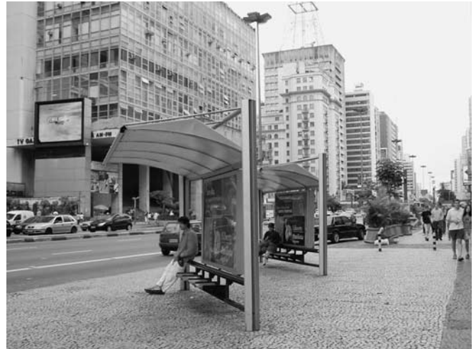
Figure 23 Angled shelters to improve customer and driver visibility.
