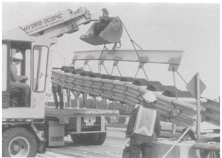
Use of preassembled low-maintenance attenuator unit saves installation time.
