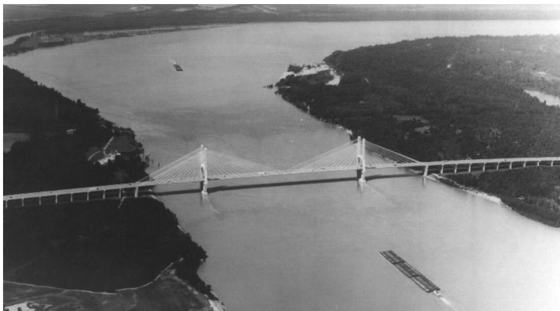
Aerial photograph of Greenville reach on Mississippi River with northbound barge traffic in foreground, existing U.S. 82 bridge removed, and sketch of new three-span cable-stayed bridge superimposed.
