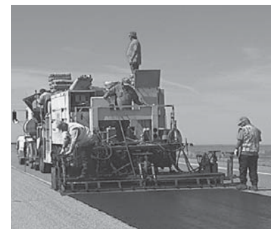
Left: Applying sealant to a flexible pavement. Right: Continuous microsurfacing, applied to high-volume, flexible-pavement roads in Michigan, fills ruts, improves skid resistance, retextures surface, and removes distortions.
