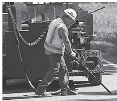
Left: Applying sealant to a flexible pavement. Right: Continuous microsurfacing, applied to high-volume, flexible-pavement roads in Michigan, fills ruts, improves skid resistance, retextures surface, and removes distortions.
