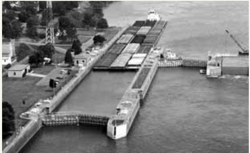
Waterborne commerce on Upper Mississippi River makes maximum use of locks that in some cases are more than 50 years old.
