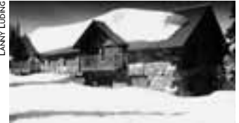
Sperry Chalet in Glacier Park, built by Great Northern Railway.
