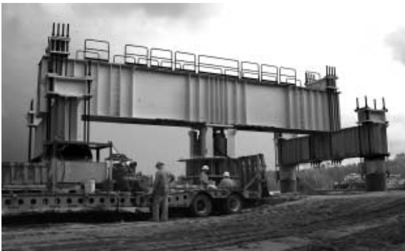
Caltrans crew applies 8-million-pound load to test pile at Santa Clara River Bridge, U.S. 101.
