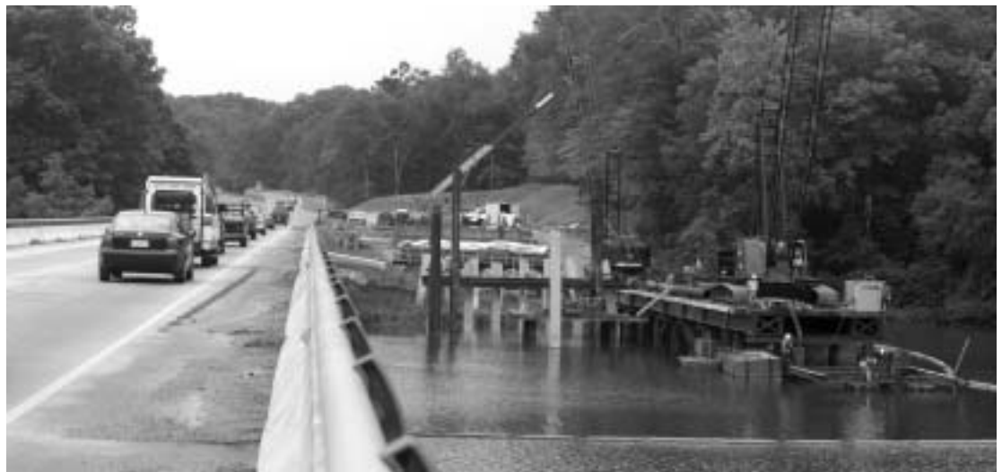
Bridge widening (above, on VA-199) is an aspect of capacity expansion.
