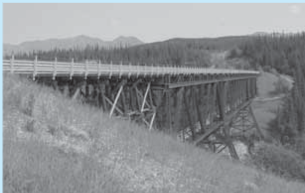
Bridge on McCarthy Road in Alaska preserves the rugged but environment-friendly ideals of the neighboring communities.
