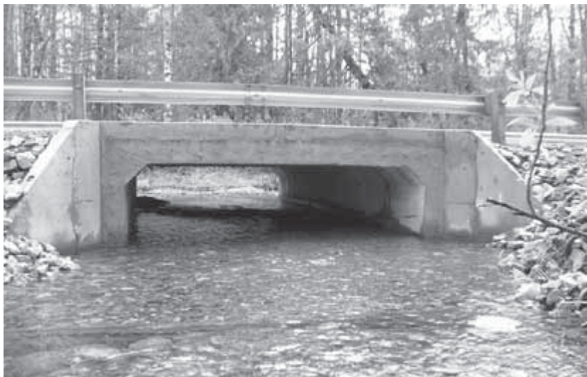
Washington State DOT has procedures to remove fish passage barriers during road construction and routine maintenance of failing culverts.
