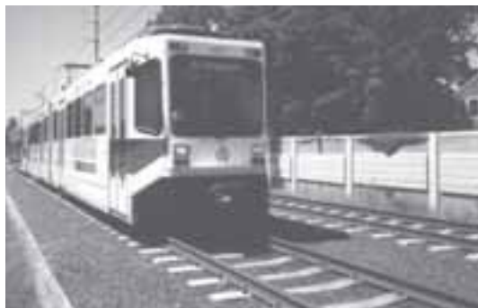
Sound-absorbing wall shields residences from noise generated by Portland TriMet transit rail.
