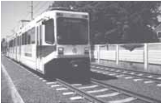
Sound-absorbing wall shields residences from noise generated by Portland TriMet transit rail.
