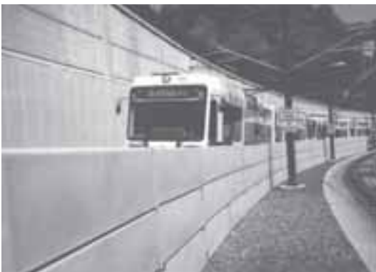
Portland TriMet transit rail passes between a sound-absorbing wall and a sound barrier wall.
