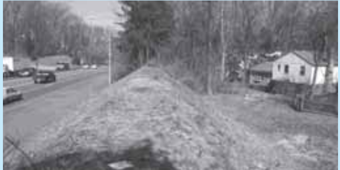
Berm construction is generally preferred by builders.
