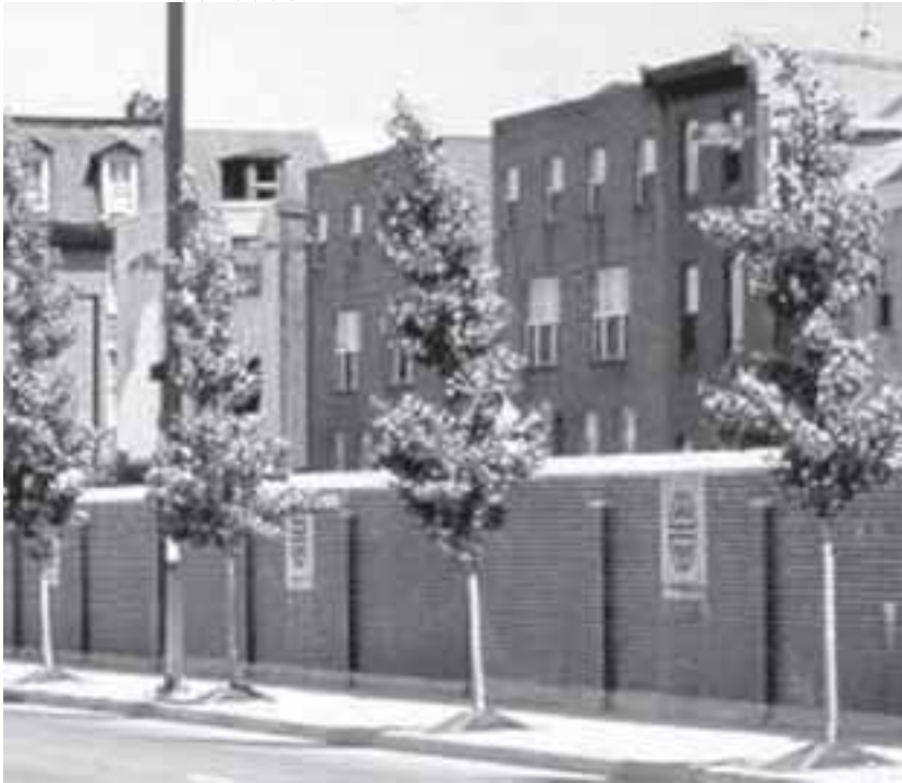
Sound barrier wall on urban street.
