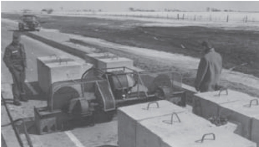
Above, left: Mechanical oscillator on a bridge. Above, right: Vibrating truck on bridge.
