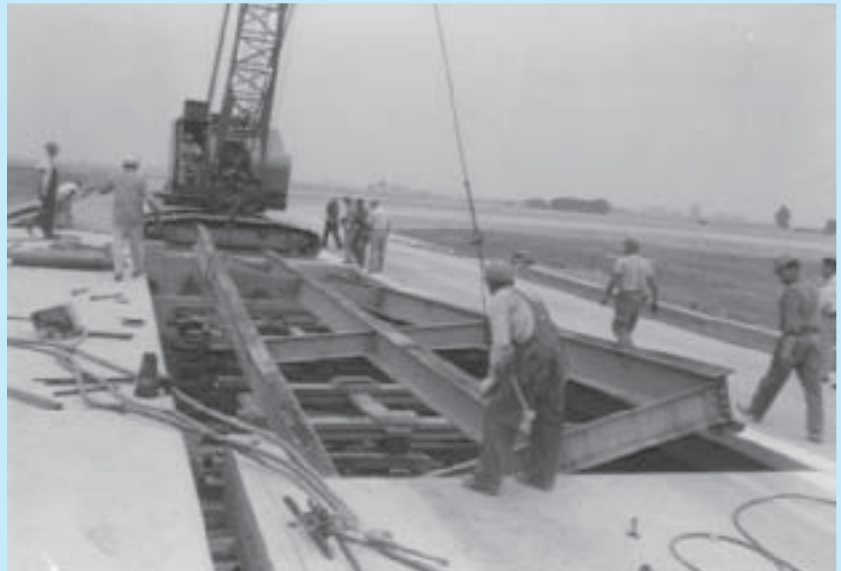
Removing damaged steel from test bridge.
