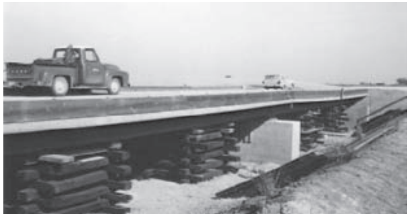
Cribbing placed below test bridges.
