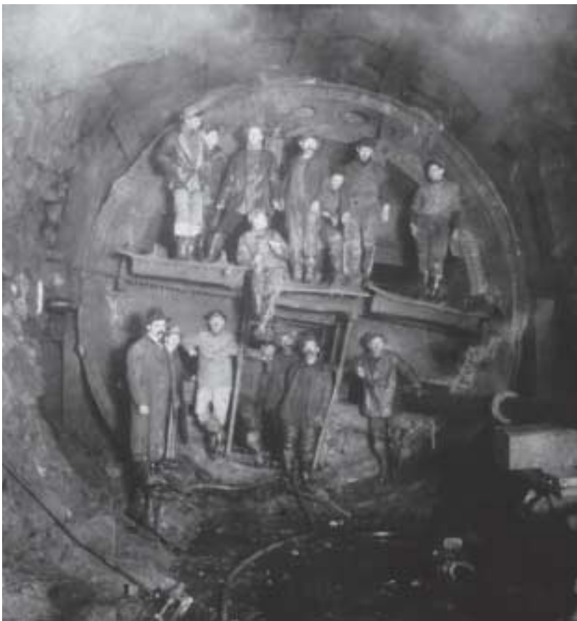
Digging out the Steinway Tunnel below the East River, to connect Manhattan and Queens by subway.
