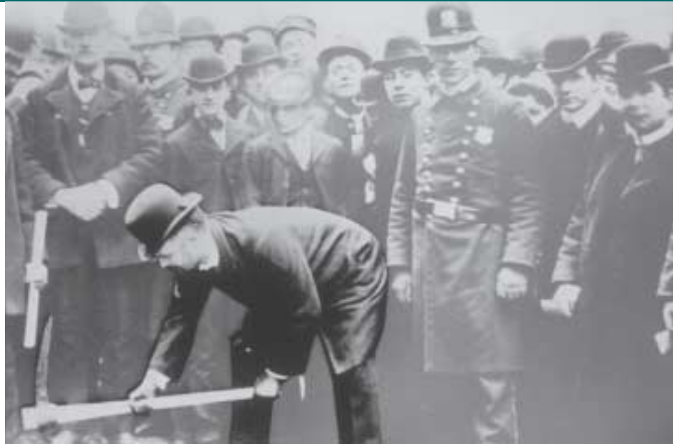
Parsons swings the pickax to start construction on the subway at Bleecker and Greene Streets.
