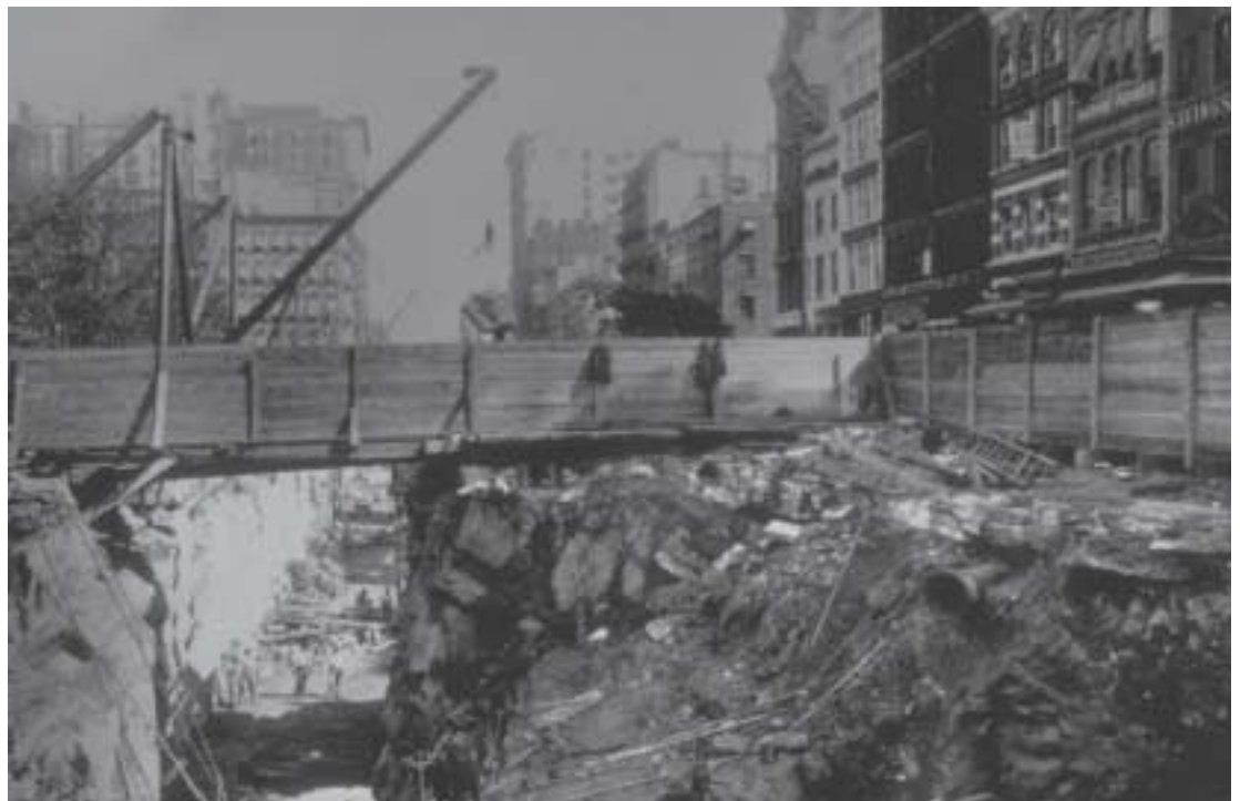
Cut-and-cover construction of the subway earned the name "Parsons's ditch."
