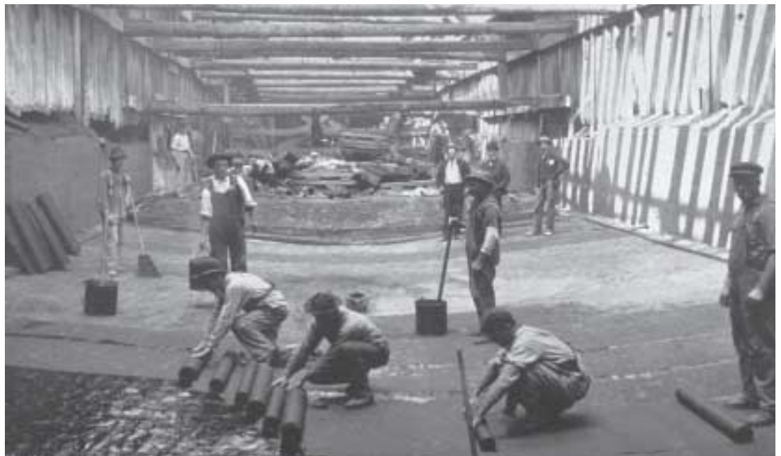
Workers at 149th Street and Courtlandt Avenue in the Bronx, September 1902.
