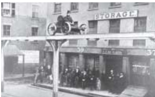
Charles T. Harvey, who designed and promoted the West Side and Yonkers Patent Railway, runs a test on Greenwich Street, 1867. The system experienced frequent breakdowns and closed in 1870.
