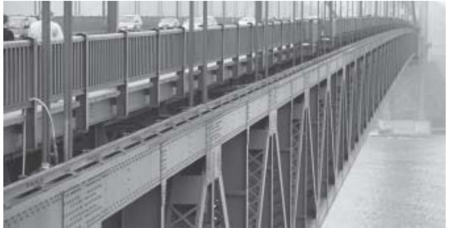
The Golden Gate Bridge between San Francisco and Northern California took 4 years to build; Golden Gate Strait below is 400 feet deep, and the bridge's two towers rise 746 feet.
