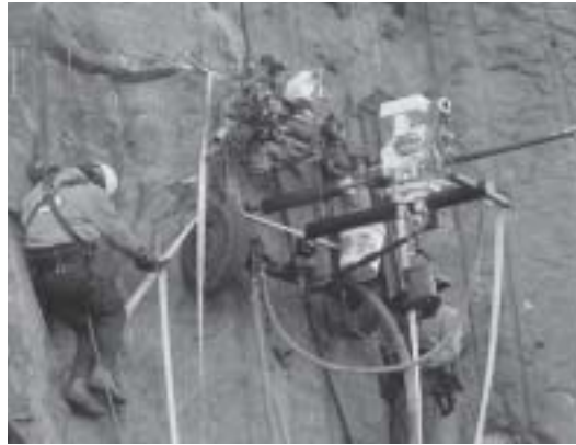
Overcoring to exhume rock reinforcement.
