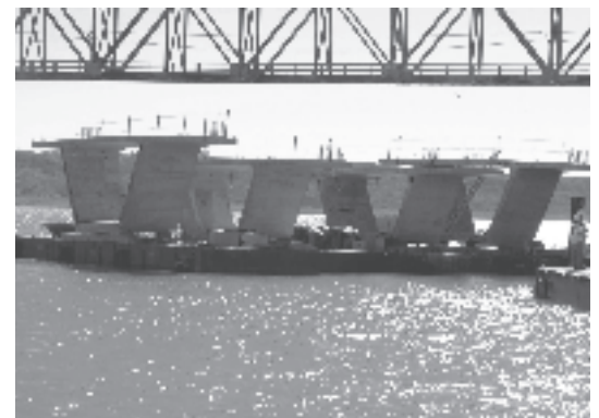
The west segment of Pier 2 of the new bridge is lifted into position ( above ). Cantilever segments arrive via barge ( below ).
