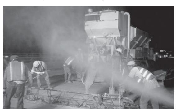
Placing an LMC-VE overlay with conventional equipment. The concrete is batched and mixed in a mobile concrete mixer and struck off with a vibrating screed. A fog spray is applied, as shown, to increase the relative humidity and help prevent plastic shrinkage cracking.
