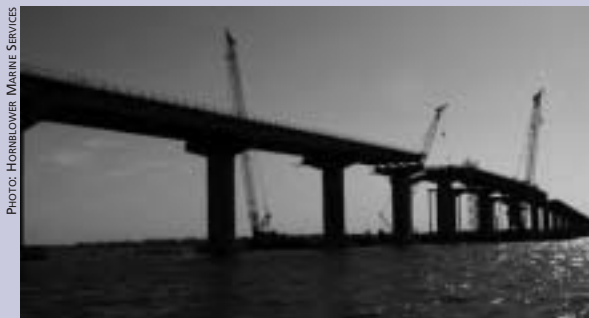
Remnants of the I-90 bridge (left) in Bay St. Louis, Mississippi, after Hurricane Katrina in August 2005, and the new bridge nearing completion in spring 2007.
