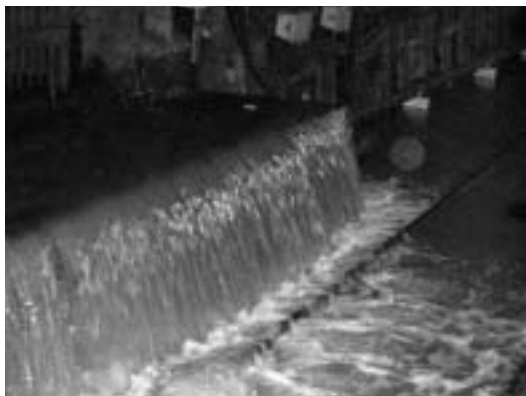
(Left:) Floodwaters at an interchange station pour over the platform into a subway tunnel after a break in the wall separating two subway lines. (Right:) During the 2002 floods, rail seals failed to withstand the hydrostatic pressure after the tunnel gates were locked; water gushed through into the next section of the tunnel.
