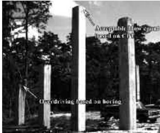
FIGURE 2 Pile Driving on the I-310/US 61 Interchange near New Orleans
