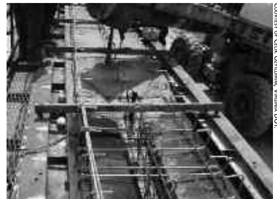
Self-consolidating concrete during placement.
