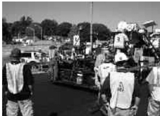
Demonstration of warm-mix asphalt paving ( left ). Warm-mix asphalt mixtures can be manufactured at production facilities with reduced emissions and decreased energy use.
