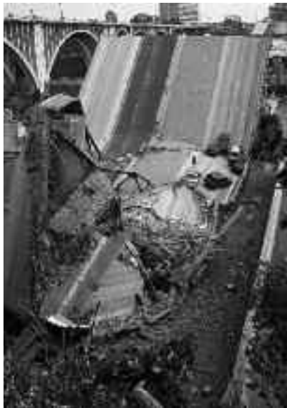
Steel-truss bridge on Interstate 35, Minneapolis, Minnesota, after collapse, August 1, 2007.
