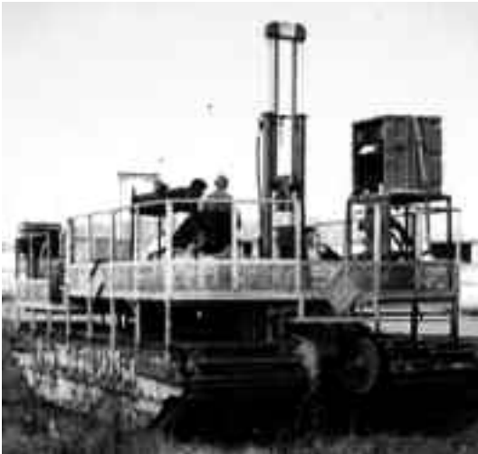
CPT testing on South Louisiana marsh deposits.
