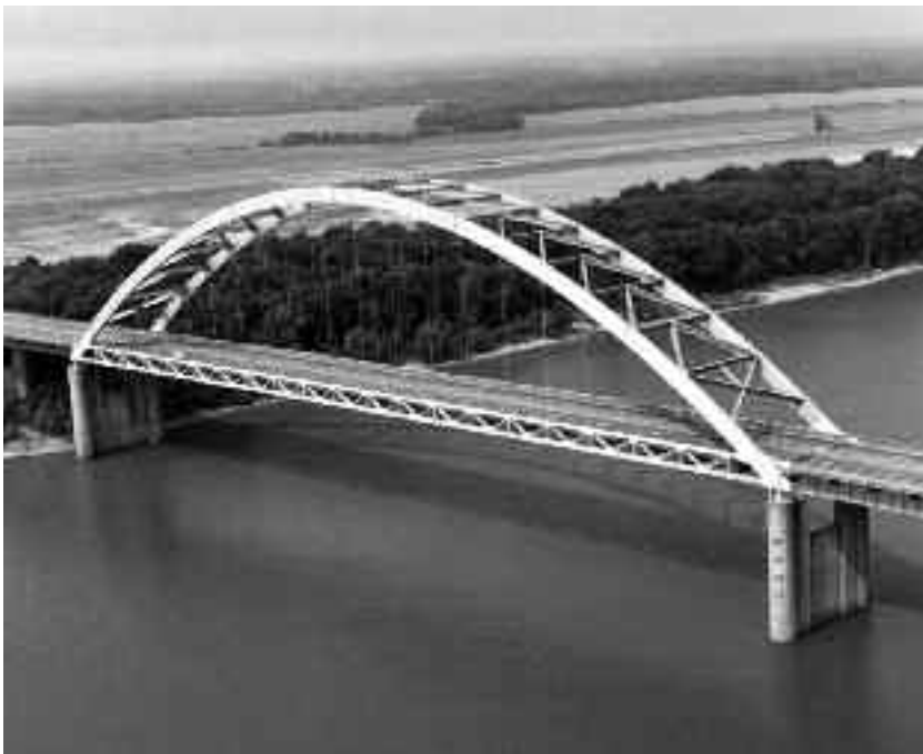
Strain gauges, accelerated monitoring equipment, and finite element modeling were combined for major design retrofit of fatigue-cracked arch ties on the FAI 24 Bridge crossing the Ohio River between Illinois and Kentucky.
