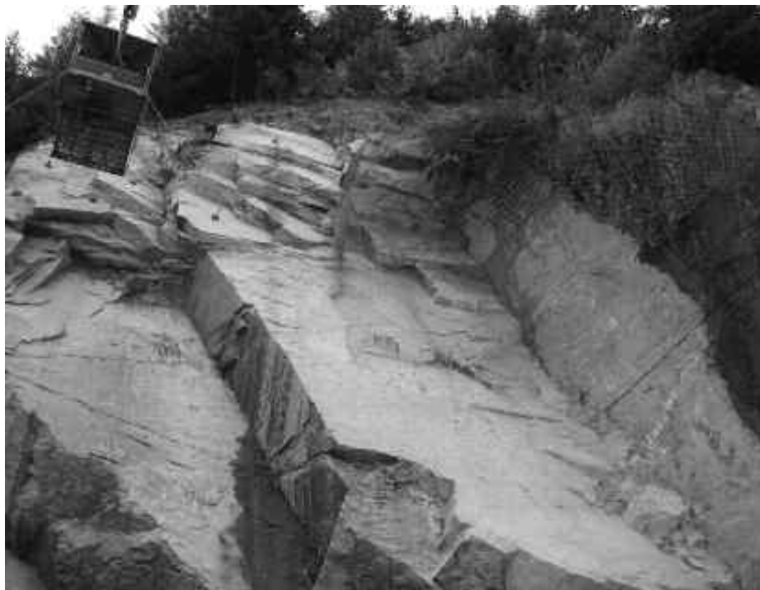
A rock fall–prone slope is scanned to determine structural soundness.
