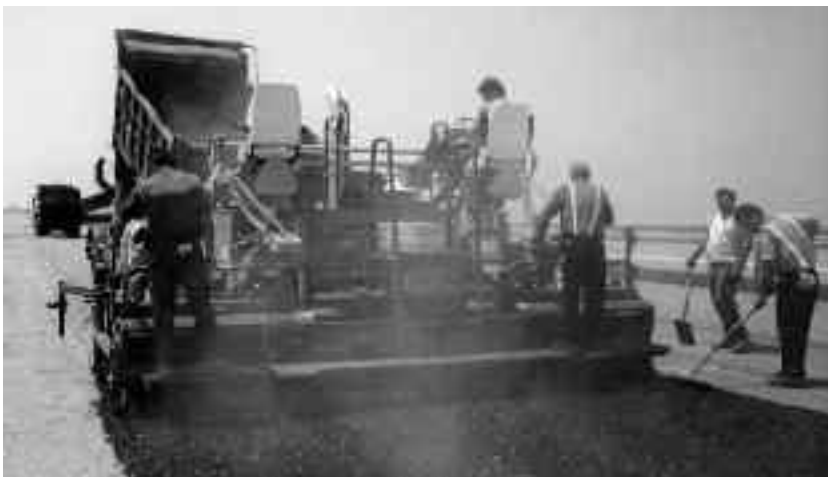
Asphalt mix is applied to a roadway; developments are sought in materials and techniques to increase service life and cost-effectiveness, as well as environmental compatibility.
