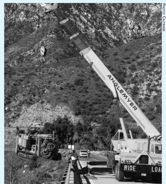
A California Department of Transportation bridge rehabilitation project on Route 39.
