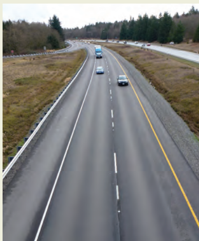
Old concrete panels beneath I-5 in Washington State caused severe cracking in the roadway (top). Washington State DOT piloted a web-based decision support tool for in-place pavement recycling and seated the concrete with an asphalt concrete overlay (bottom).
