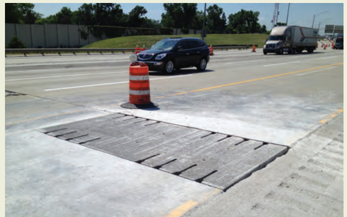
A precast panel in place on the northbound Tri-State Tollway near Roosevelt Road, Illinois Route 38.
