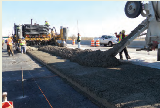
A concrete ready-mix truck wind-rowing concrete for the top lift of a composite pavement in front of a single-lane slip-form paver on the Reagan Memorial Tollway.
