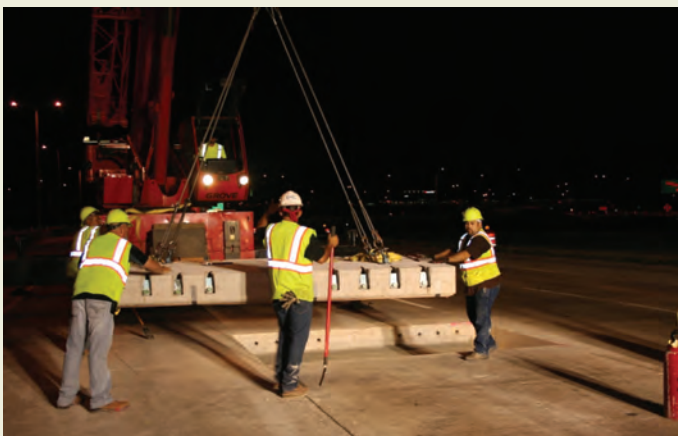
Crews place a precast panel on the central Tri-State Tollway, Interstate 294.
