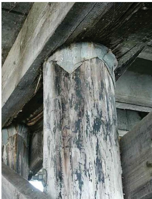
A timber cap abutment has collapsed onto a timber piling as a result of decay and bearing loads.
