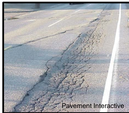
Inadequate compaction results
