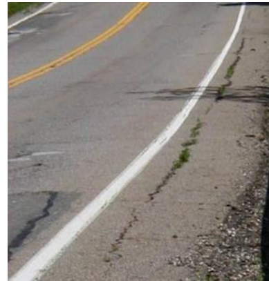
Figure 4.3-7 - Left: High Severity Transverse Pavement Cracks, Right: High Severity Longitudinal Pavement Cracks
