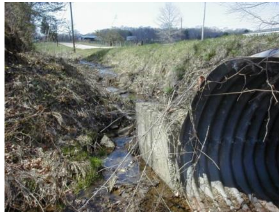
Figure 4.4-3 – Minor Rill from Roadway Runoff
