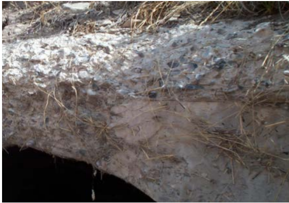
Figure 4.10-7 – Severe Freeze-Thaw Deterioration with Stand-Out Aggregate and Pop Outs
