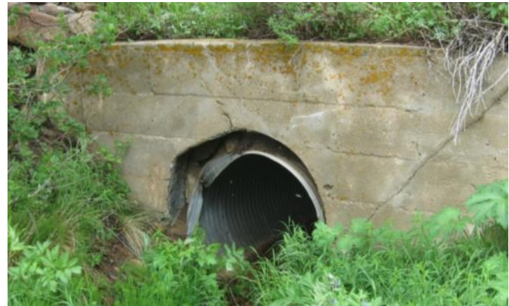
Figure 4.6-5 – Separation of Headwall and Culvert Pipe
