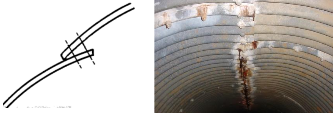
Figure 4.15-1 – Cocked Seam with Cusp Effect
