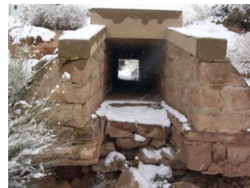
Figure 4.7-5 – Severe scour undermining wing wall foundation
