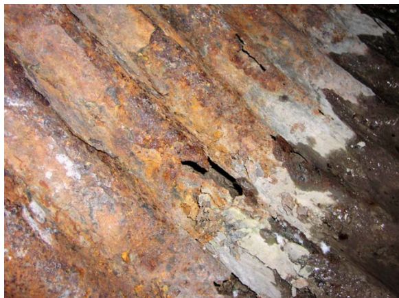
Figure 2.3-1 – Severe Corrosion of Corrugated Steel Pipe
