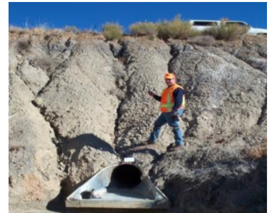
Figure 4.4-4 – Severe Gullying with Severe Sheet Erosion
