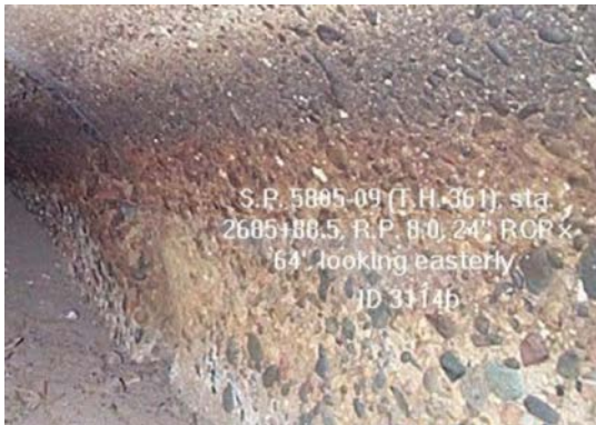
Figure 4.10-8 – Moderate Deterioration (Probable Chemical Attack) with Exposed Aggregate and Loss of Surface Mortar
