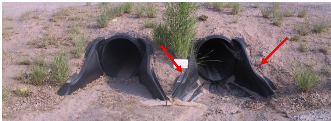
Figure 4.6-4 – Deformation of Prefabricated End Sections
