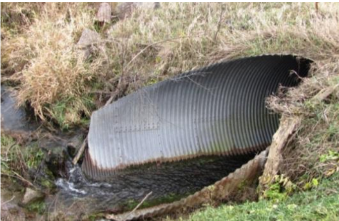
Figure 4.6-2 – Erosion Around Mitered End Section (Photo shows erosion on sides and below mitered end section)
