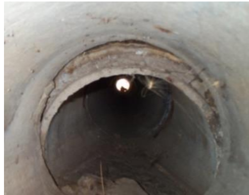
Figure 4.14-7 – Joint Offset Causing Completely Dislodged Pipe Section
