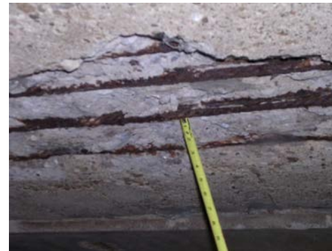
Figure 4.10-4 – Left: Small Spall along Crack, Right: Large Spall with Exposed/Corroded Rebar
