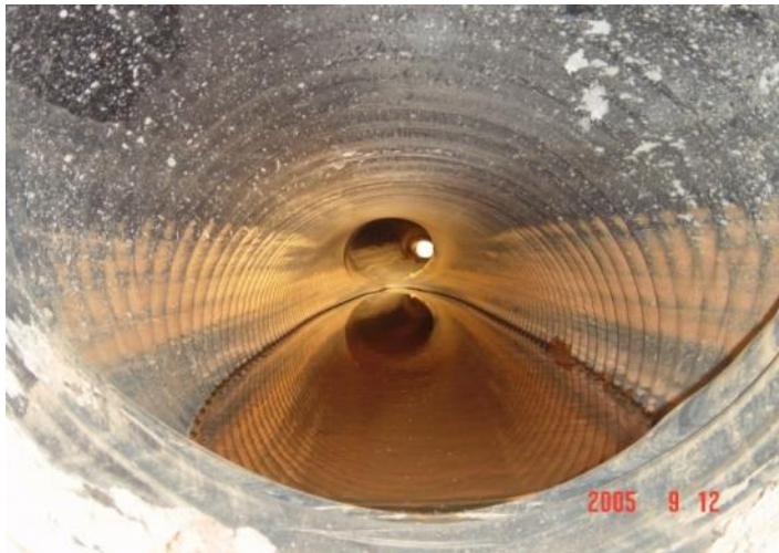
Figure 4.8-1 – Severe visible sag in vertical alignment causing ponding
