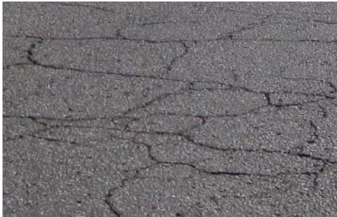
Figure 4.3-8 – Alligator Cracking in Pavement
