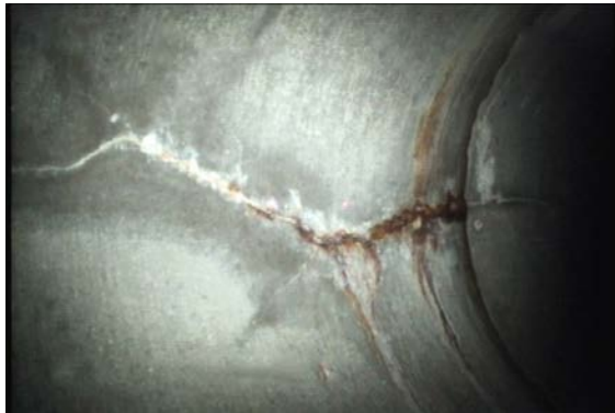
Figure 4.10-2 – Pipe with Critical Longitudinal Cracks with Rust Staining and Efflorescence
