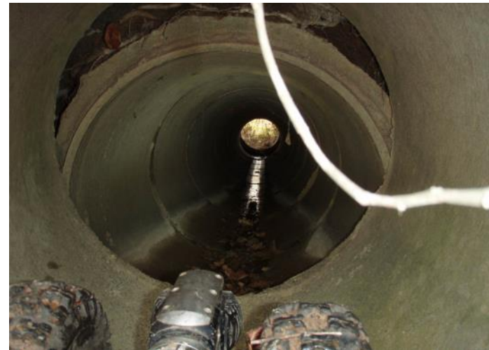
Figure 4.8-2 – Severe vertical misalignment has dislodged pipe segment resulting in joint offset and loss of support to embedment soil
