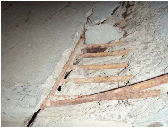
Figure 2.3-3 – Corrosion of Reinforcing Steel in Concrete Pipe
