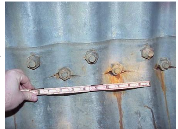
Figure 15-3 - Cracking at bolt holes
