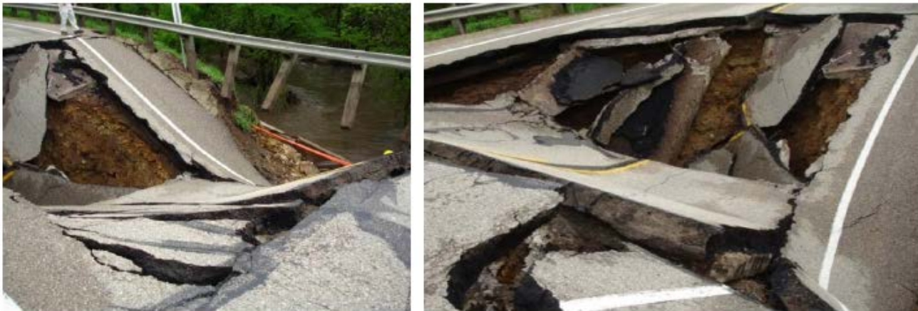
Figure 1.2-3 – Roadway Collapse Due to Structural Failure of Culvert (Photo courtesy of Iowa Department of Transportation)
