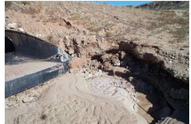
Figure 4.5-2 – Bank erosion adjacent to culvert
