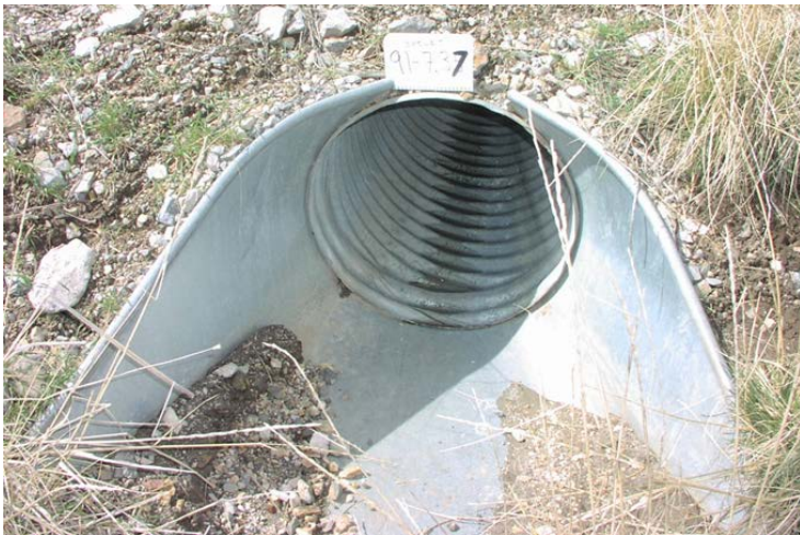
Figure A.3-5 – Apron (also called Flared End Section) on Corrugated Metal Pipe
