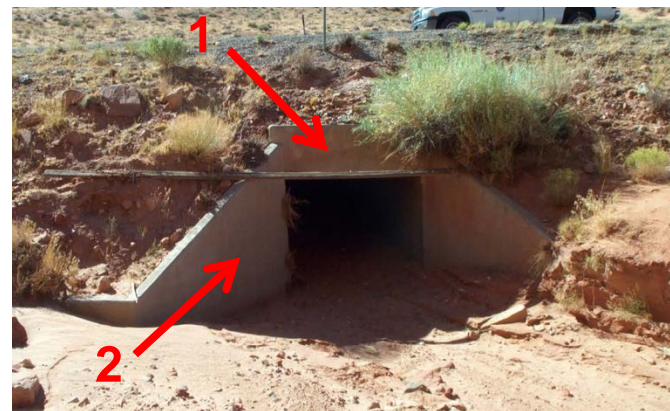
Figure A.3-6 – Headwall (Arrow 1) and Wingwall (Arrow 2) on Concrete Box
