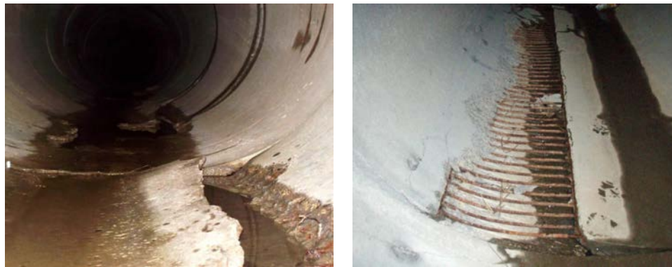
Figure 4.10-6 – Slabbing in concrete pipe
