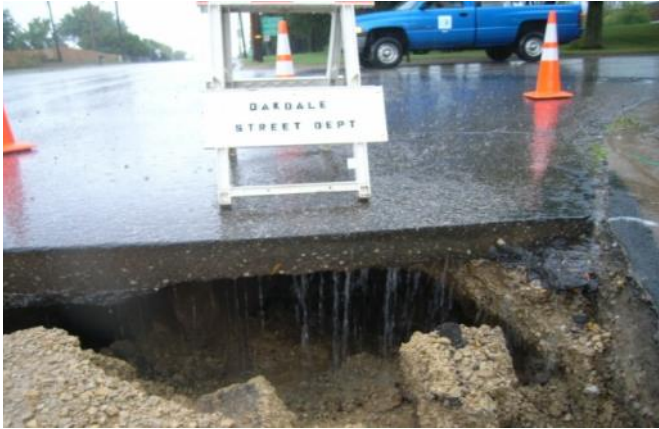
Figure 4.3-5 - Bridging in Flexible Pavements
