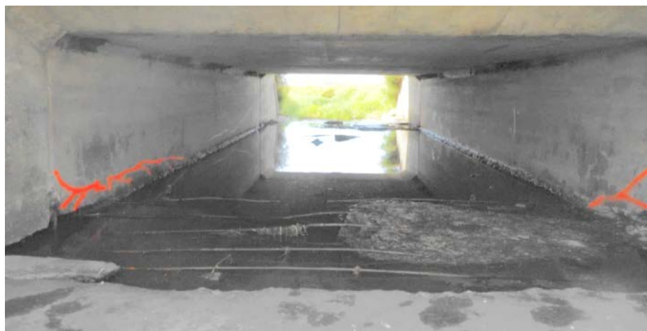
Figure 4.7-6 – Invert slab in critical condition due to severe degradation of concrete
