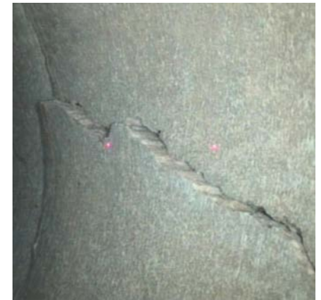
Figure 4.10-3 – Cracks with Radial Offset
