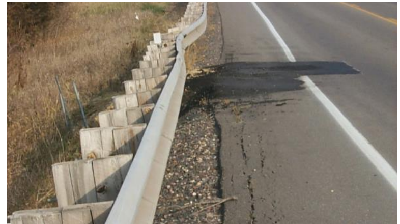
Figure 4.3-9 - Misalignment of Guardrail at Culvert Outlet (Note also patching of pavement, cracking and sagging at same location)
