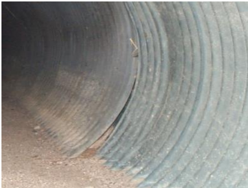
Figure 4.14-6 – Joint Separation in Corrugated Metal Pipe with Visible Backfill
