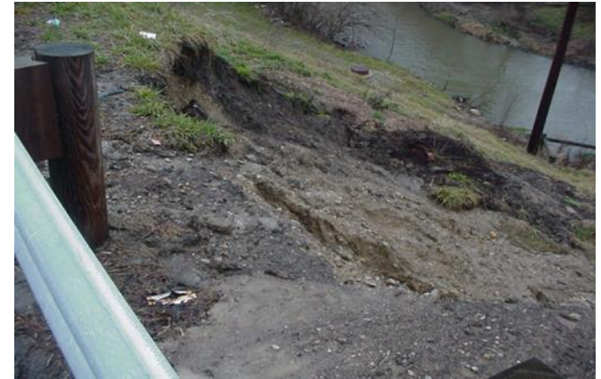
Figure 4.4-1 - Embankment Sloughing
