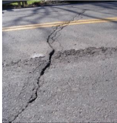
Figure 4.3-7 - Left: High Severity Transverse Pavement Cracks, Right: High Severity Longitudinal Pavement Cracks
