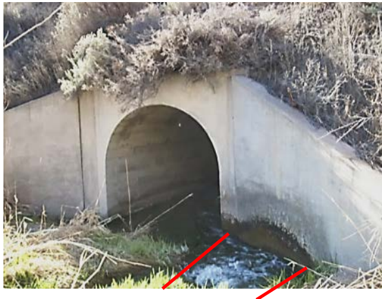
Figure 4.5-1 – Change in stream alignment causing flow to be directed into wingwall
