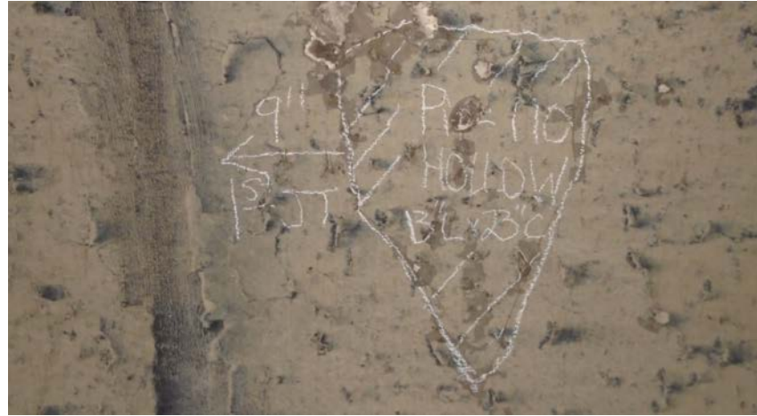
Figure 4.10-5 – Delaminated Area Marked on Pipe Wall, Located by Sounding with Hammer
