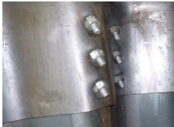
Figure 4.15-2 – Severe Bolt Tipping in Corrugated Metal Plate
