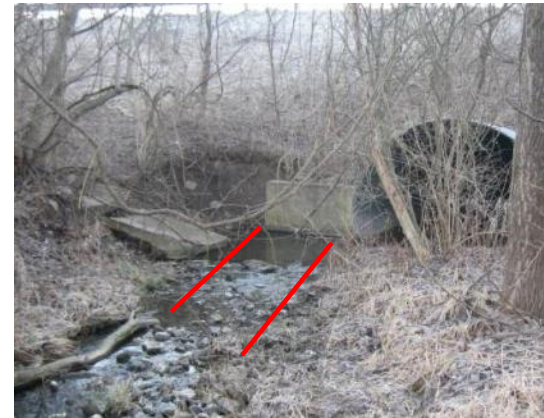
Figure 4.5-1 – Change in stream alignment causing flow to be directed into wingwall
