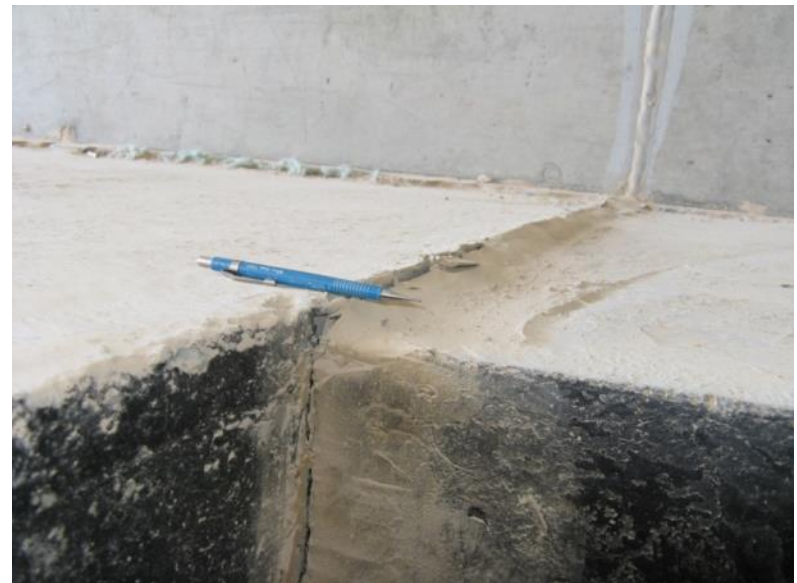
Figure 4.7-2 – Differential Settlement of Footing Supporting Corrugated Metal Arch
