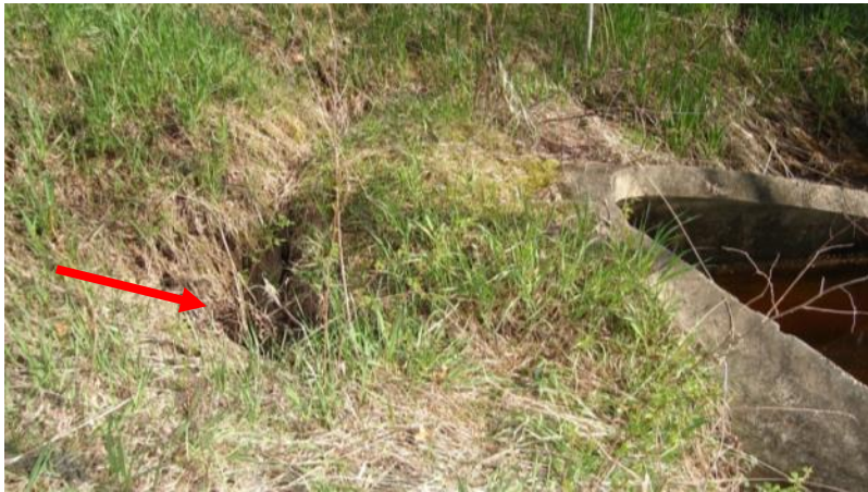
Figure 4.6-3 – End section drop-off due to erosion under projecting end
