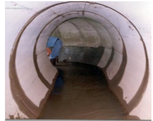
Figure 4.14-9 – Water Infiltration through Joints
