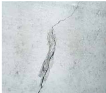
Figure 4.10-4 – Left: Small Spall along Crack, Right: Large Spall with Exposed/Corroded Rebar
