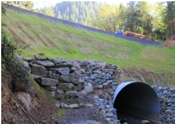
Figure 4.4-2 – Moderate Sheet Erosion on Steep Embankment
