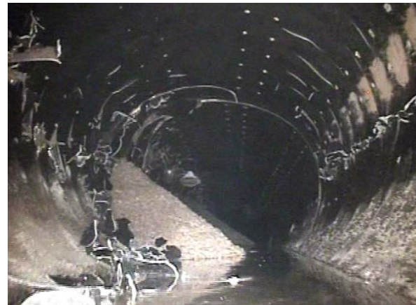
Degradation and Cracking of HDPE Pipe
