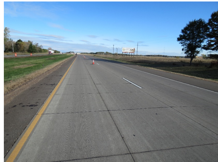
Lower volume interstate (6" thick) BCOA
