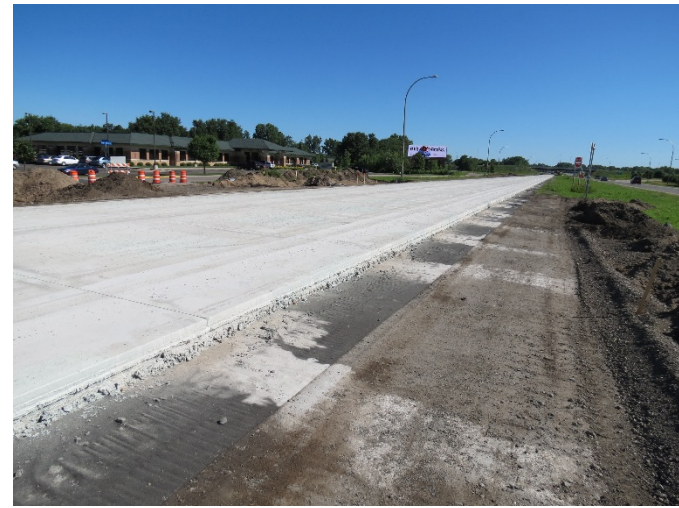
State highway (6" thick) UBOL
