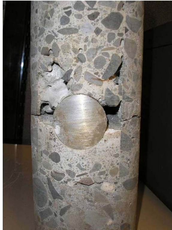
Backfill material consolidation
