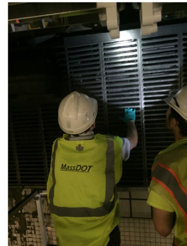
Photo 7. Checking wall grating and panels for stability
