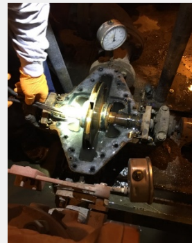
Pump Obstruction Removal
