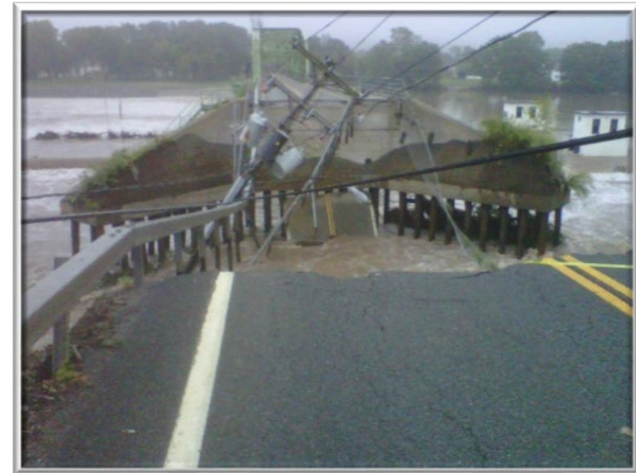
Hurricane Irene Damage, 2011
