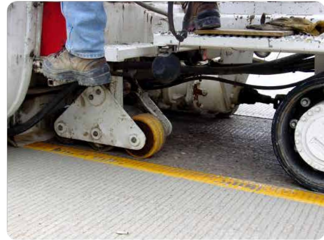
Proper Slurry Recovery System
