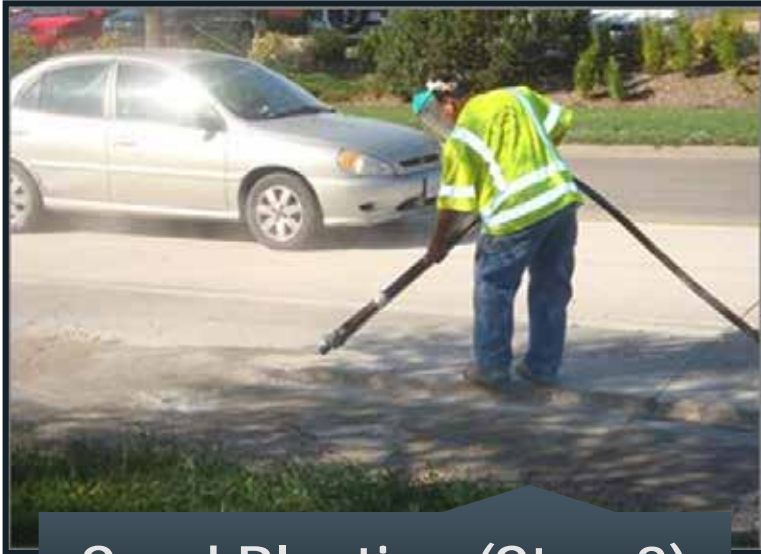
Sand Blasting (Step 3)
