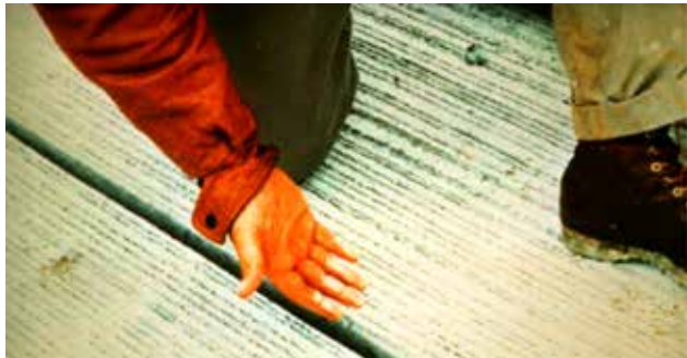
Joint preparation (=clean & dry!)
