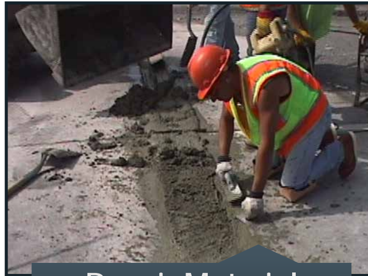
Repair Material Placement (Step 6)
