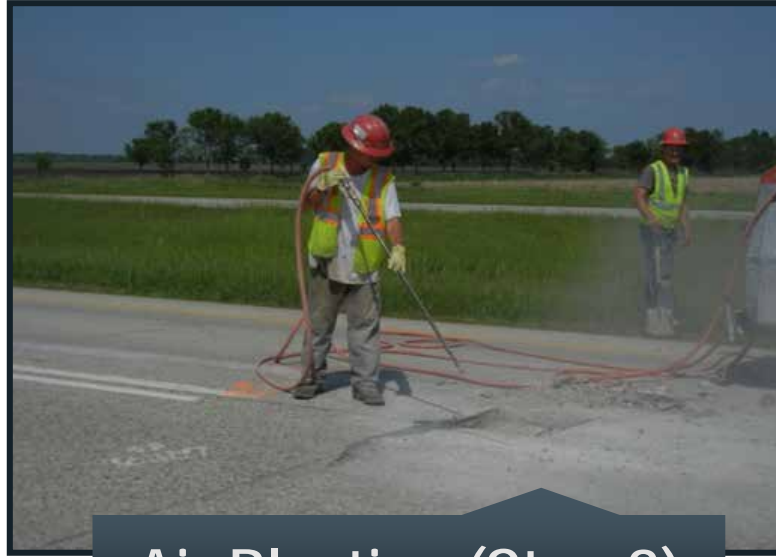
Air Blasting (Step 3)
