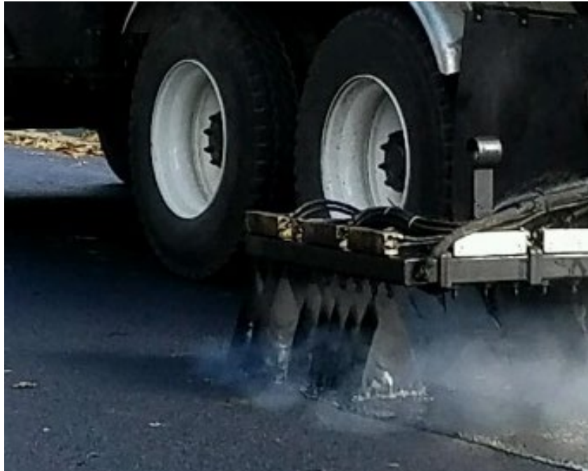
Hot-applied treatment – under the joint
