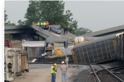
M bridge, Missouri (2013)
