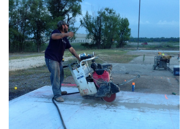
Saw Cut Joints
