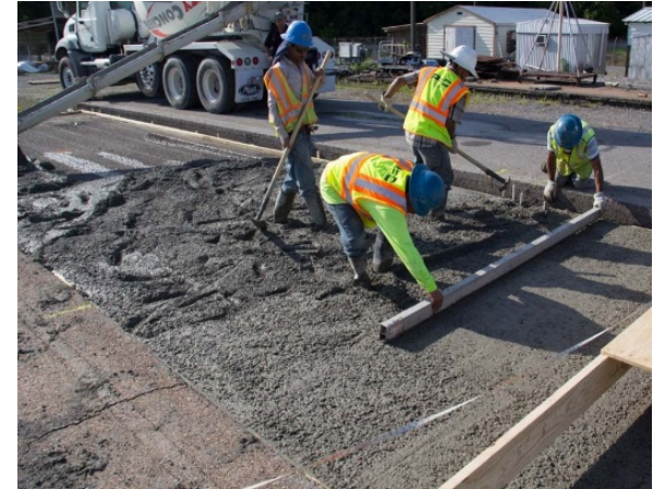
Levelling and Troweling of concrete
