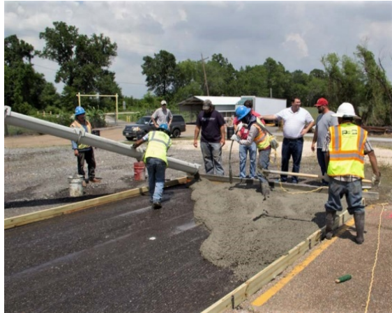
Placement of concrete overlay
