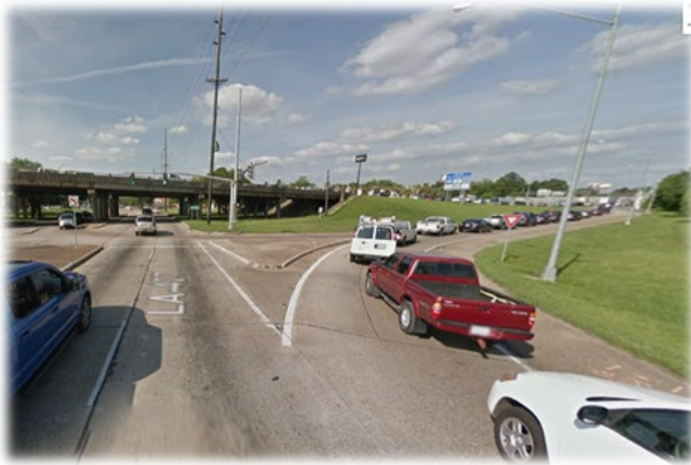
Spillback from on-ramp
