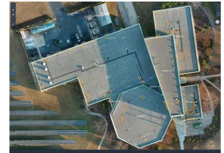
Roof Assessment (Visual)
