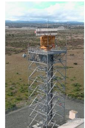
MRY ASR Radar Facility
