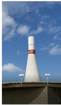
VOR Navigation Facility
