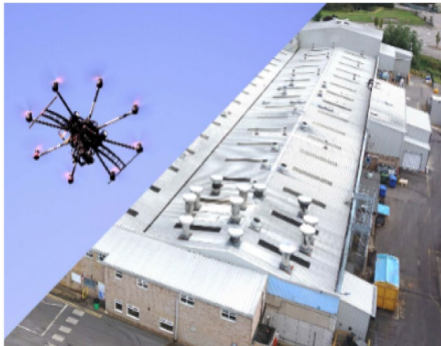
DJI Matrice UAS used for aerial roof inspection
