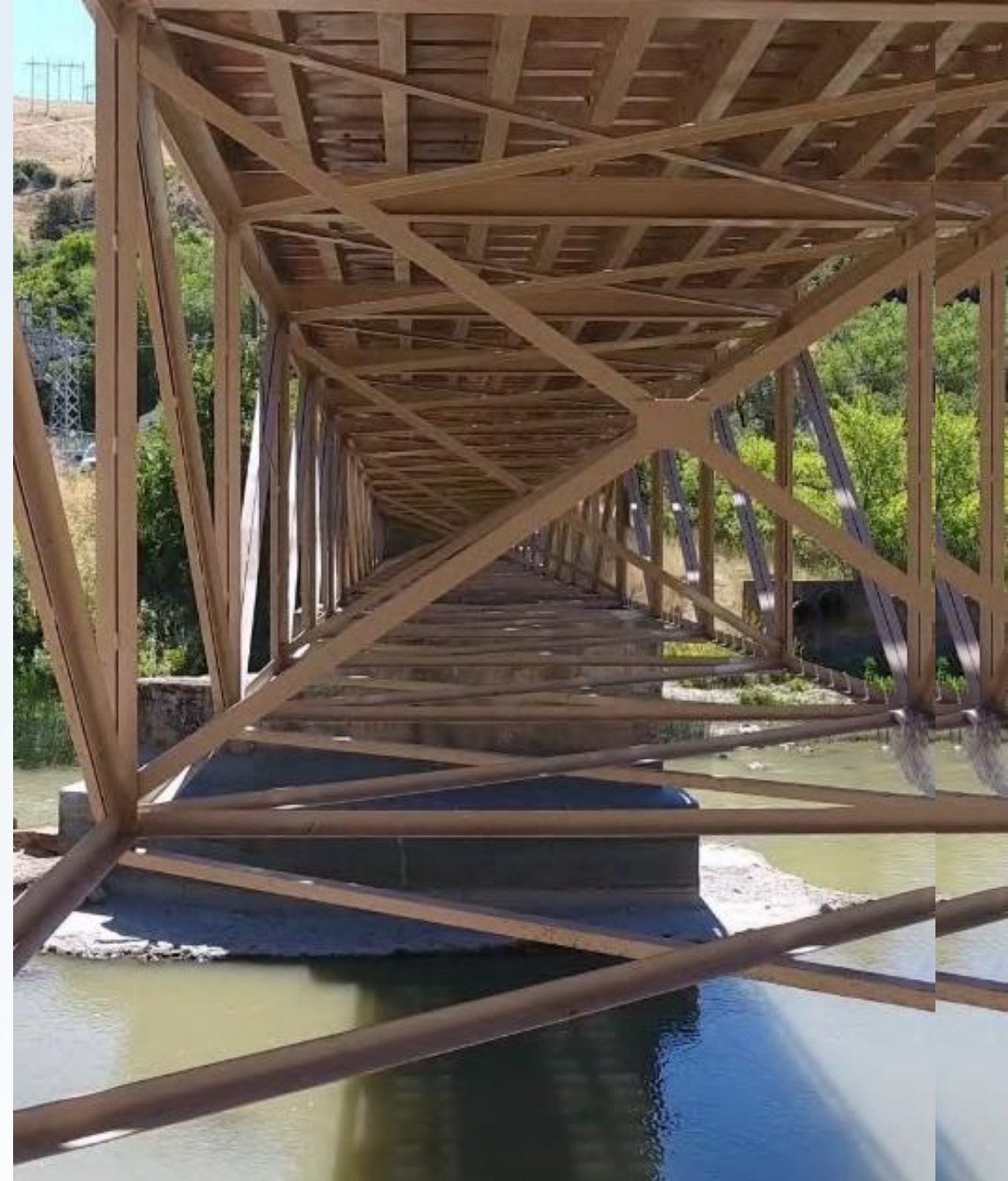
Cutler Bridge drone inspection image. Courtesy UDOT.
