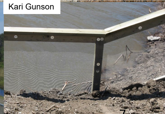
Mesh Hardware cloth (wire) with steel frame (left); wood frame (right)
