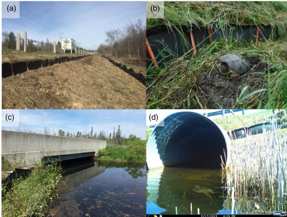
FIGURE 2 Herpetile ecopassage fence installation showing the below-grade design (a, b), and the connection to existing road crossing infrastructure (i.e., bridges (c) and culverts (d))
