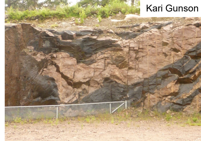
Fence-end tie-in with cliff face
