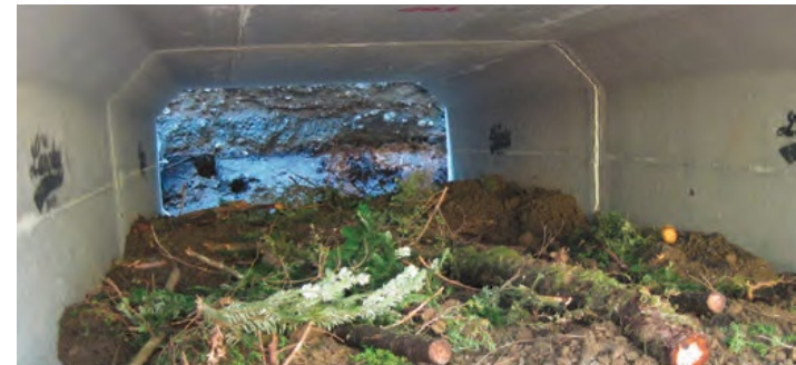
Substrate scooped into culvert (B. Beasley)
