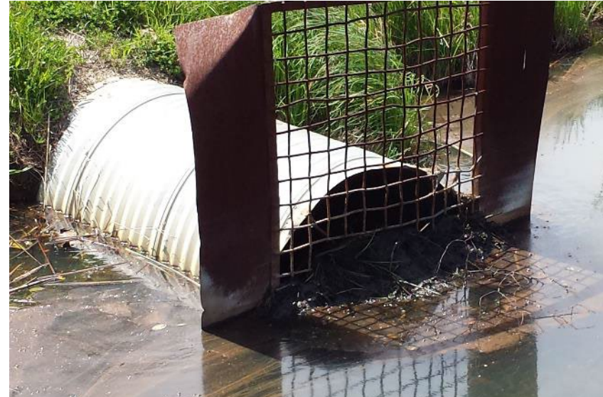
Beaver screen on existing drainage culvert, Ausable Bayfield Conservation Authority
