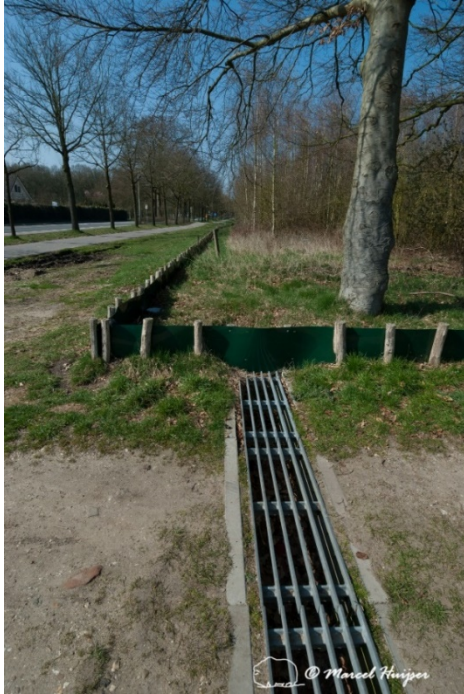
Left: A wildlife guard at a low volume dirt access road
