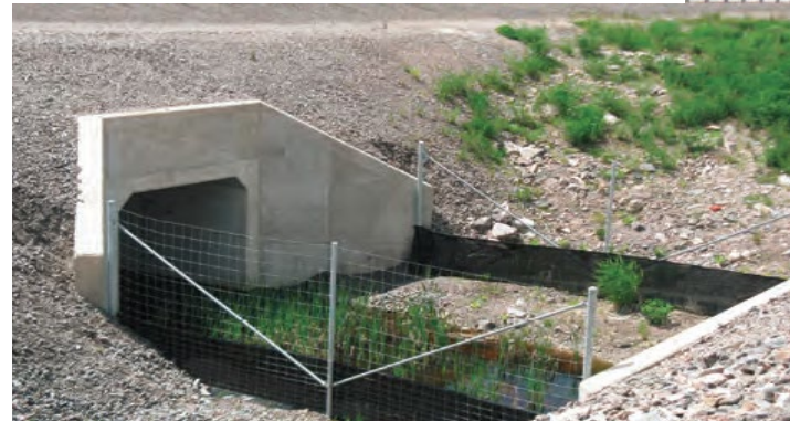
Wing walls used for reinforcement work well for wildlife (K. Gunson)
