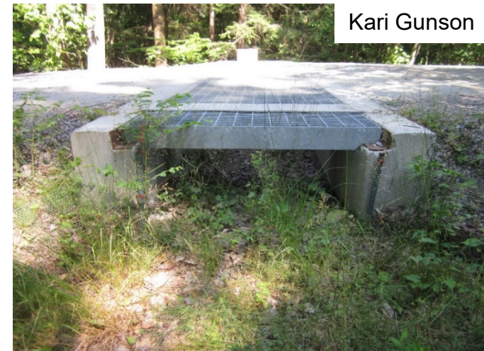
Bottom: Open-grate and open-bottom underpass, Killbear Provincial Park, Ontario
