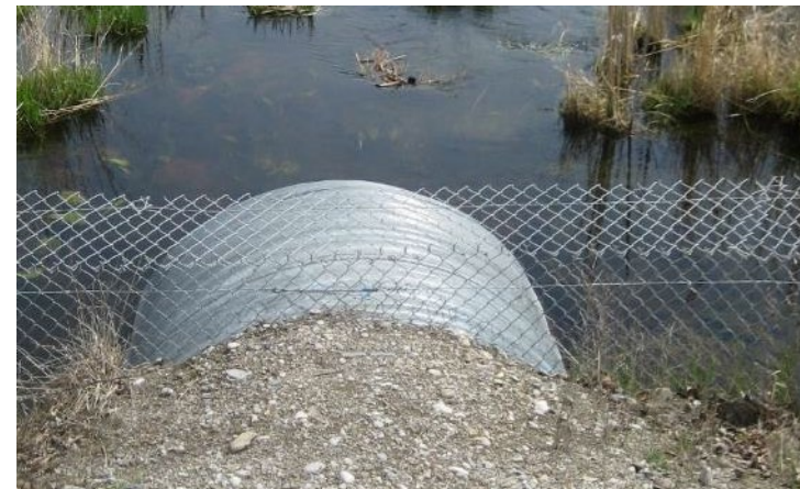
Non-designated round CSP culvert (Kari Gunson)
