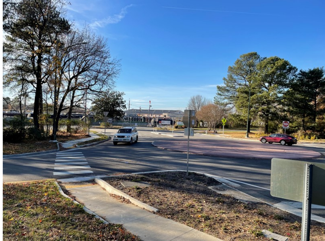
Performing well after one year traffic
