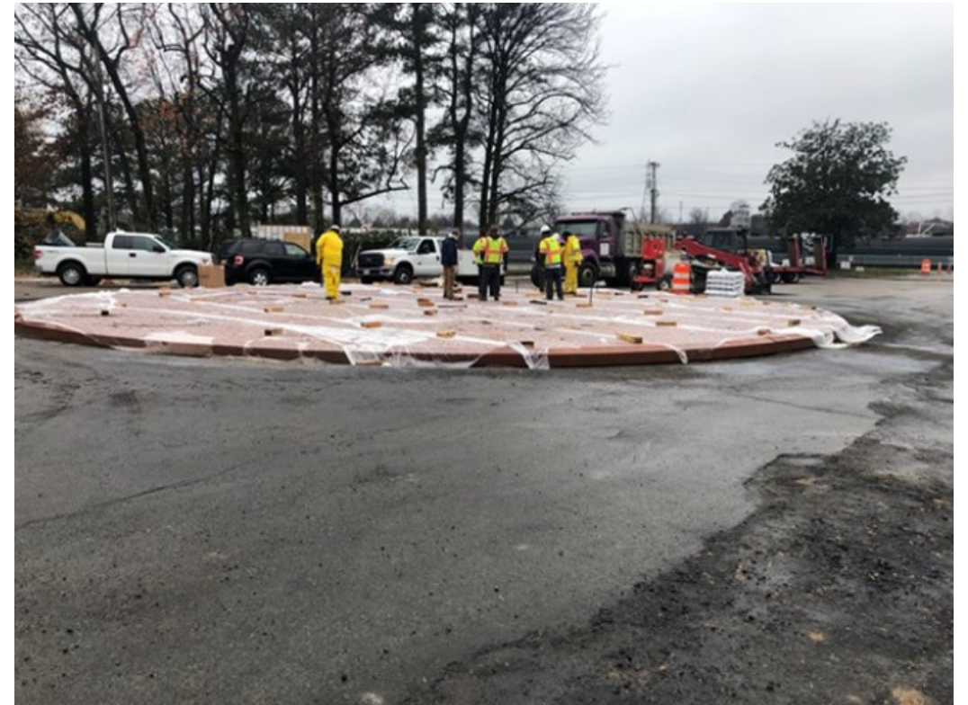
Panels for truck apron in place
