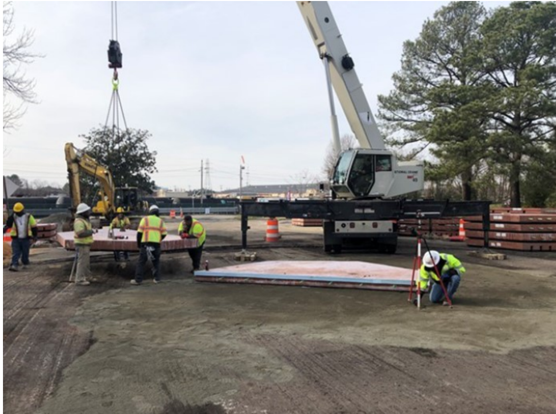
Installation of median panel
