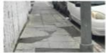
4. Cracked/Uneven Sidewalks
