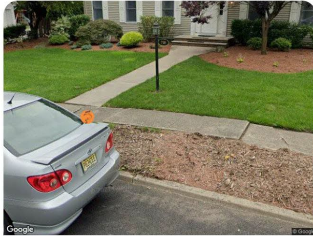
Surface Problem Severity ● ● ○ ○ ○ ○ Tags cracks
