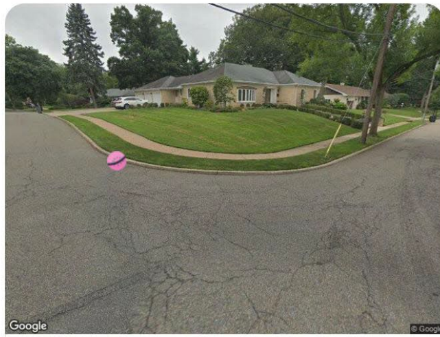
Missing Curb Ramp Severity ●●●●●● Tags no alternate route
