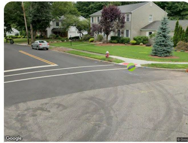
Curb Ramp Severity ●○○○○○
