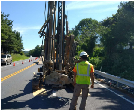
Standard Penetration Testing
