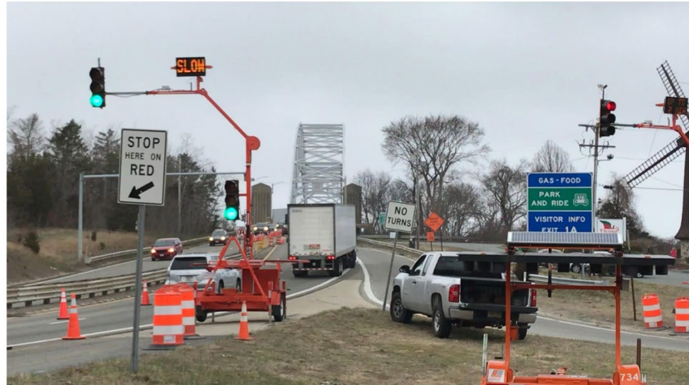
Dynamic Ramp Meter at Sagamore Bridge
